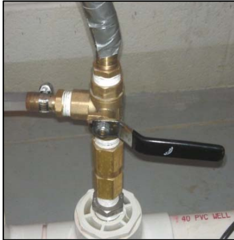
Figure 3.5 Injection line flow control valve
