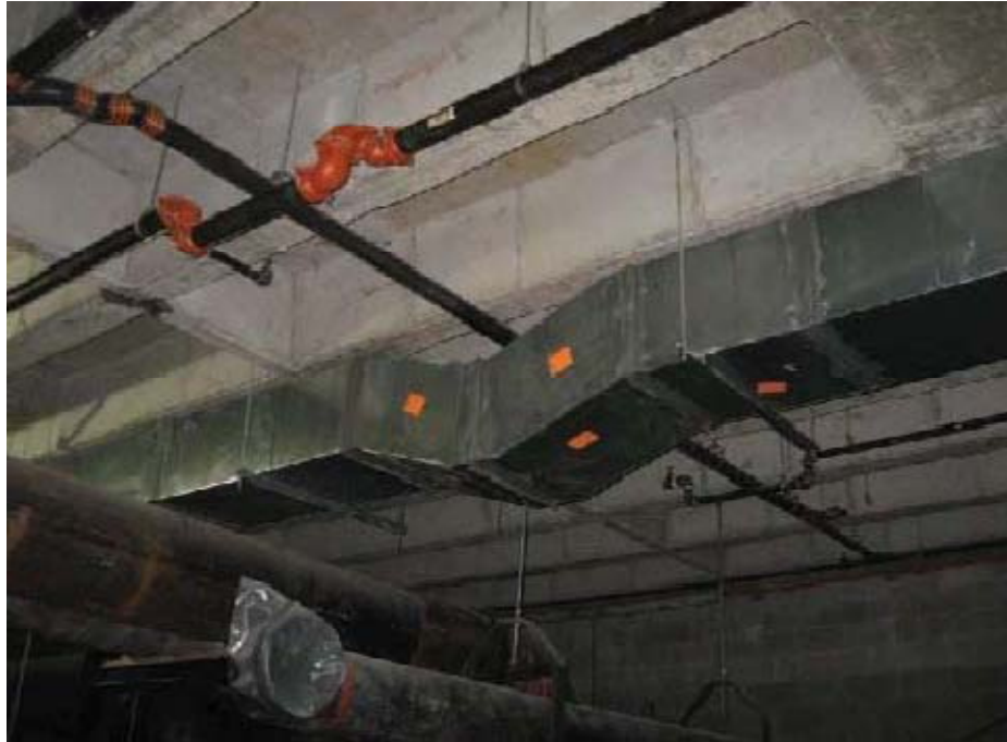
Figure 7.24: Good Coordination among Plumbing, HVAC and Concrete (Actual)
