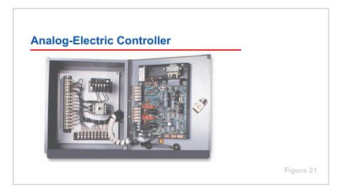
**Analog-electric** control systems vary the electric current or voltage to operate the controlled devices. A sensor sends an electric signal to the controller, and the controller sends an electric signal to operate the controlled device.
