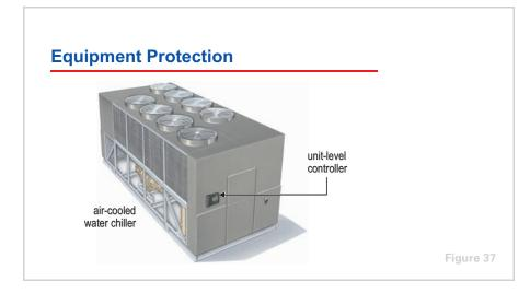
As described earlier, another important function of a unit-level controller is to protect the equipment from damage. As an example, Figure 37 shows an air-cooled water chiller with a microprocessor-based unit controller. Suppose a condenser fan motor fails during hot weather. With less air flowing through the air-cooled condenser, the temperature (and pressure) of the refrigerant inside the condenser gradually rises.
