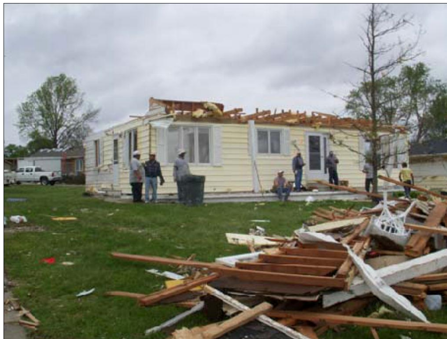
Fig. 11(b). Partially damaged example building at Parkersburg
