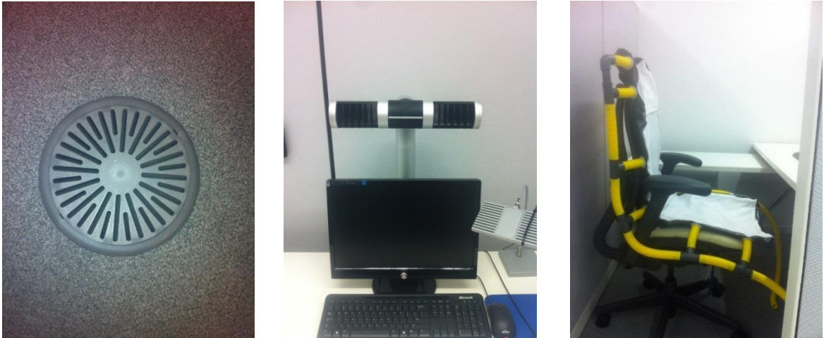
Figure 3-3 Terminal of ventilation system: UFAD (left), PV (center), CV (Right)
