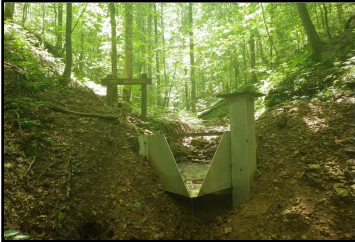
Figure 3.2: Sediment and debris buildup behind WSB flume (2016).
