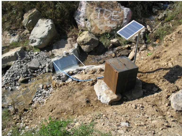
Figure 2.2: ISCO Sampler with Flume at Toe of Valley Fill A
