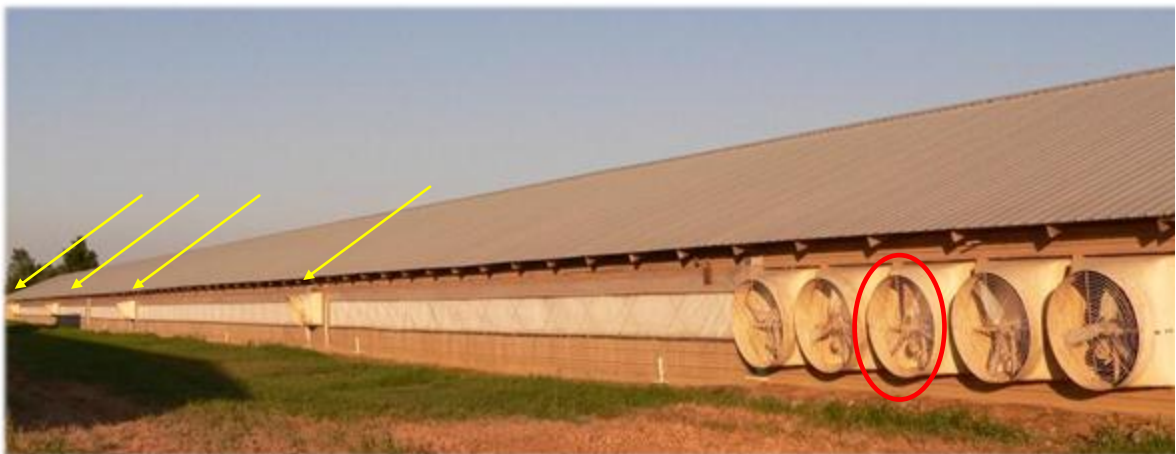
Figure 3.4. Representative barn at Farm 1 with fans placement illustrated. The circle indicates the test fan among five 1.22 m diameter Glass Pac Canada fans placed immediately next to each other. The arrows indicate four 0.91 m diameter Glass Pac Canada fans.
