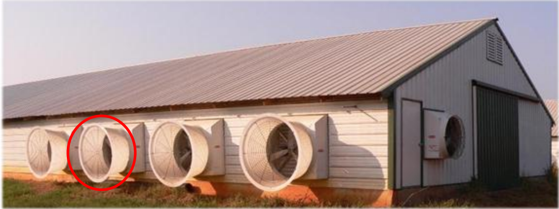
Figure 3.10. Exhaust end of a representative barn at Farm 3. Four 1.22 m diameter Chore Time Turbo fans and one 0.91 m diameter Chore Time fan. 1.22 m diameter fans were spaced 1.6 apart. Red circle indicates test fan.
