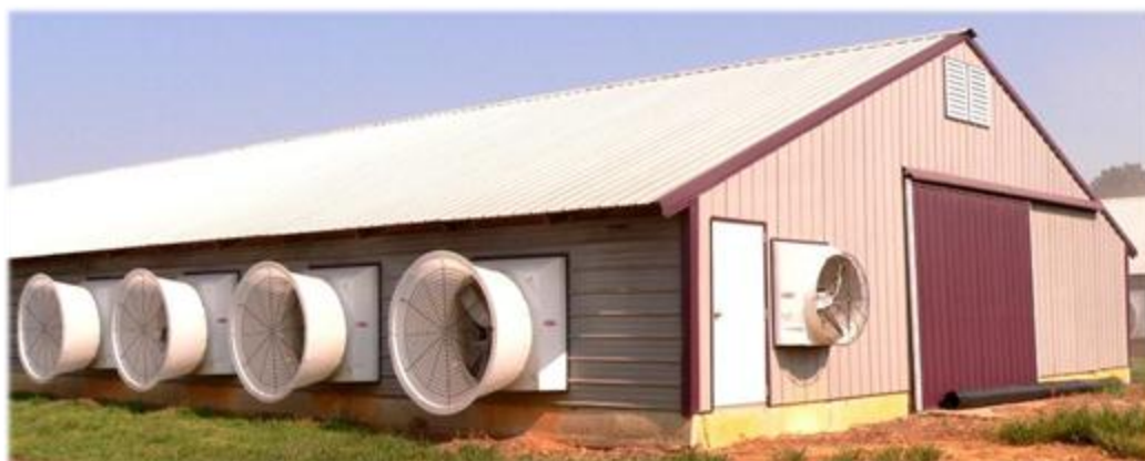
Figure 3.7. Exhaust end of a representative barn at Farm 2. Four 1.22 m diameter Chore Time Turbo fans and one 0.91 m diameter Chore Time fan.
