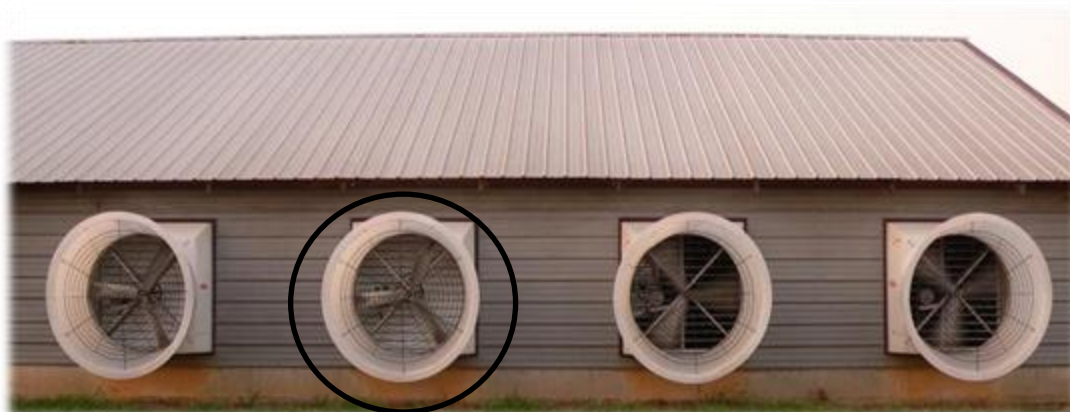
Figure 3.6. Representative barn at Farm 2 with exhaust fan placement illustrated. Fans were spaced 1.6 m from each other. The circle indicates the test fan.
