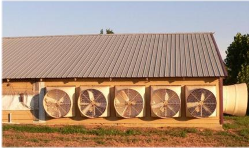
Figure 3.2. Exhaust end of a representative barn at Farm 1 with exhaust fan placement illustrated. Fans were placed immediately next to each other.
