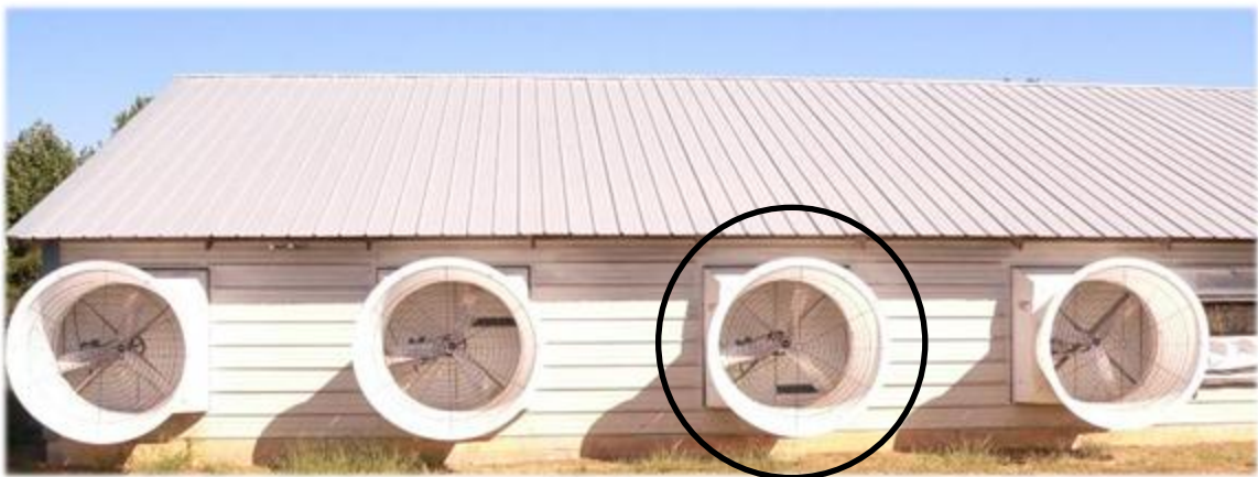
Figure 3.12. Representative barn at Farm 4 with exhaust fans placement illustrated. Fans were spaced 1.6 m apart. The circle denotes the test fan.
