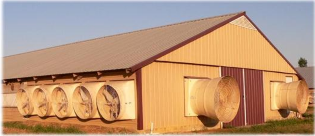
Figure 3.3. Exhaust end of a representative barn at Farm 1. Five 1.22 m diameter Glass Pac Canada fans and two 1.32 m diameter Hired Hand fans.
