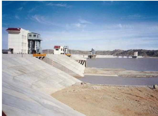
Figure 48 Project 635 in Xinjiang
