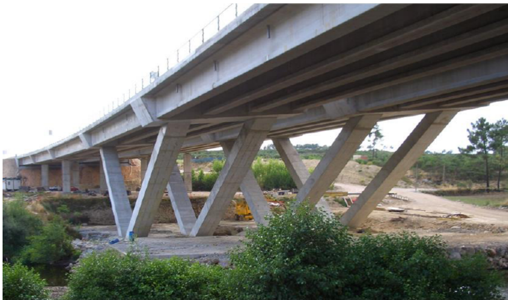
Figure 1.5 Continuous bridge with precast I-girder, courtesy D.H. Ordonez
