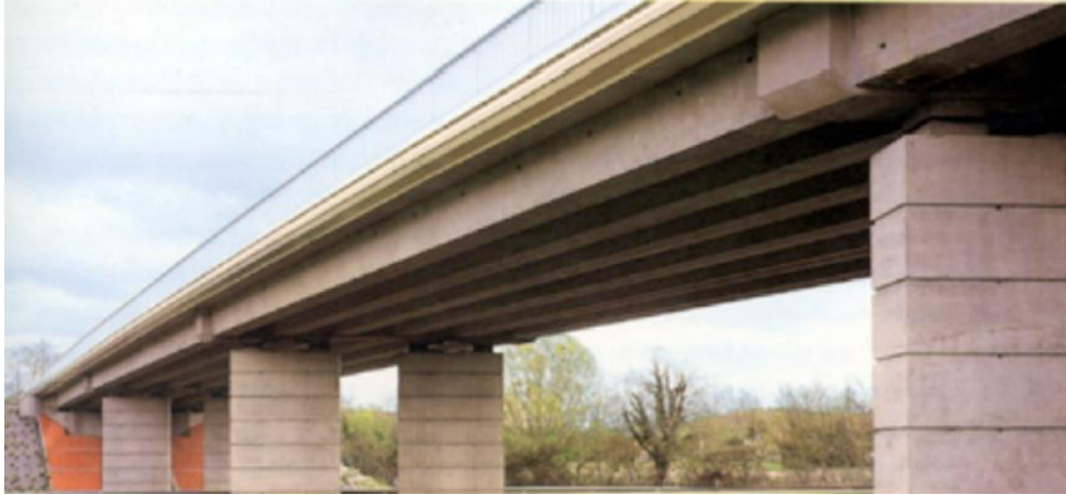
Figure 1.4 Continuous bridge with precast I-girder, courtesy D.H. Ordonez
