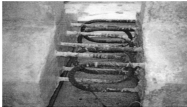
Figure 1.13 Continuity system using U-bars bent at 180°
