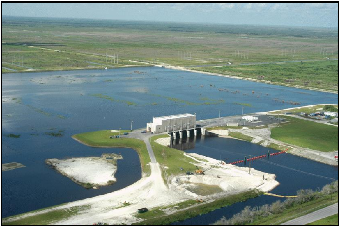
Figure 1-1 Aerial view of STA (Gonzalez, 2010)
