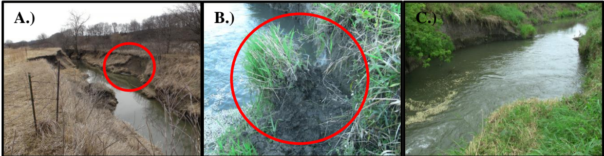
Figure 3.2: Evidence of channel degradation caused by passage of knickpoint: A.) Steep side slopes B.) Bank failures C.) Channel widening
