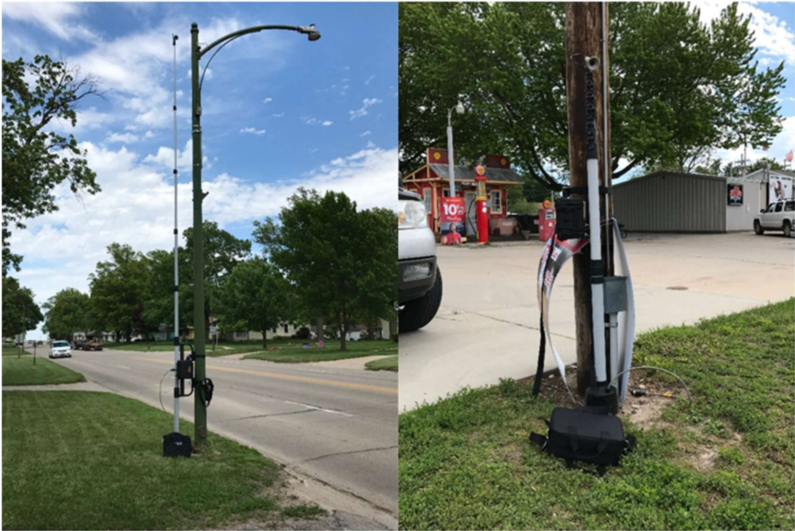
Figure 3.1 Setup of MioVision Scout cameras
