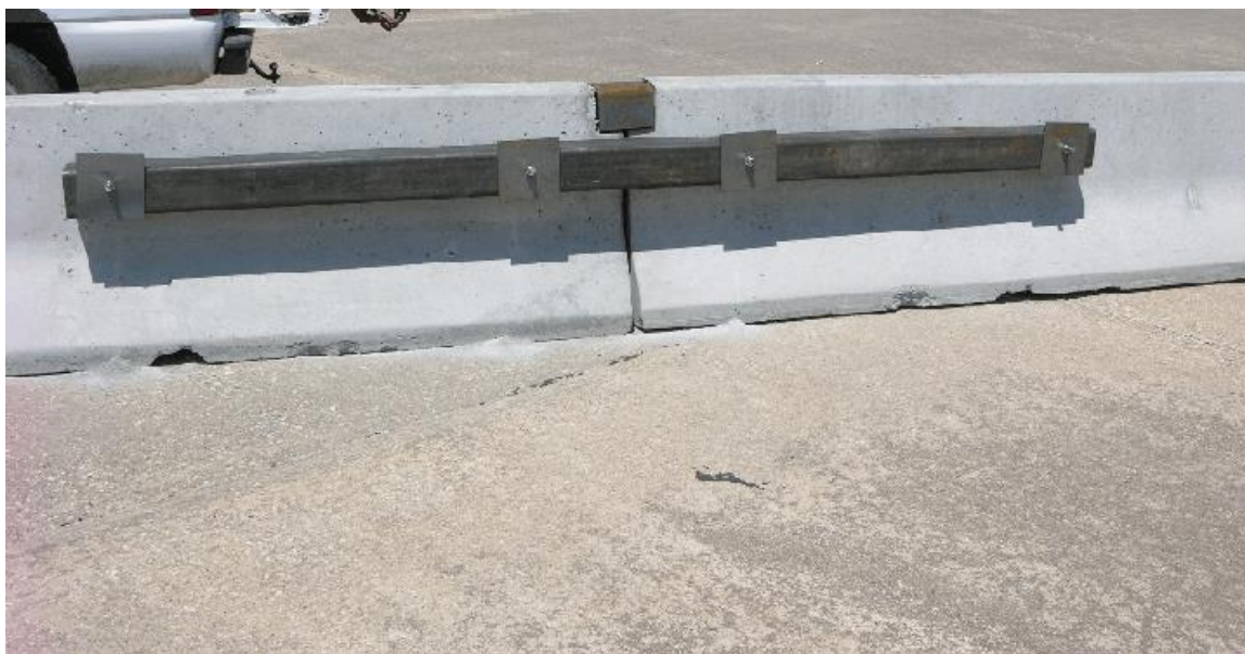
Figure 25. NYSDOT Box-Beam Stiffener System [29]
