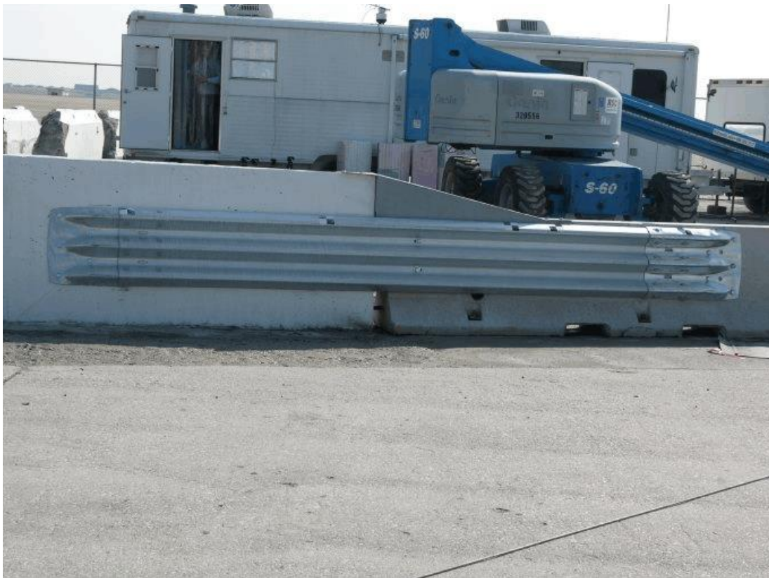
Figure 11. Transition from PCB to Permanent Concrete Barrier [2]
