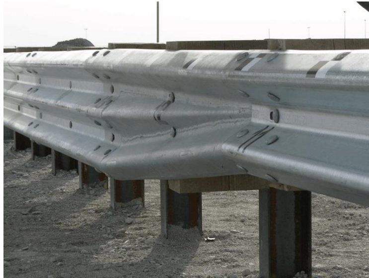
Figure 19. MGS Stiffness Transition with Asymmetrical Element [21]
