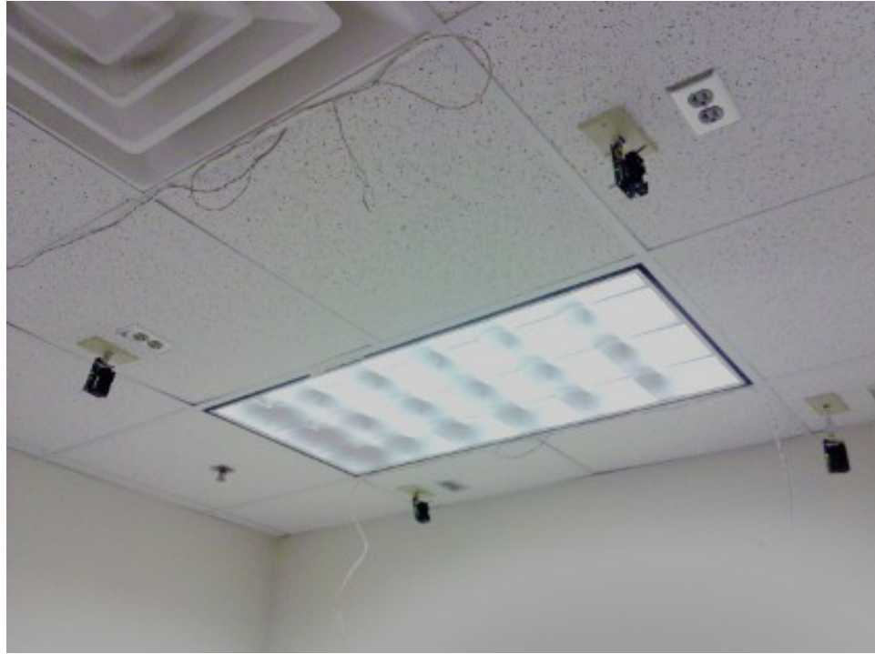
Figure 2.4: The testbed in the ceiling of the CPN Lab.
