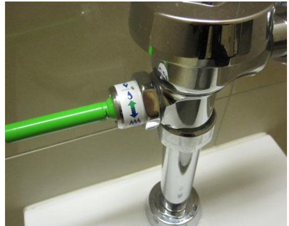
Figure 21: Sloan Uppercut ® , as installed in Columbia City Hall 2
