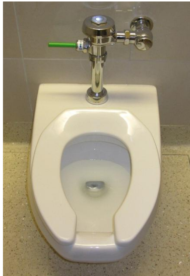
Figure 20: Sloan Uppercut ® , as installed in Columbia City Hall 1
