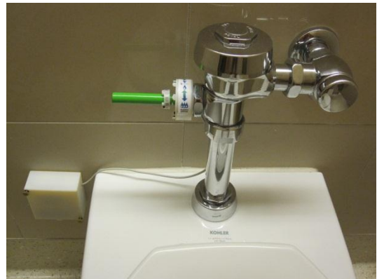
Figure 25: Flush counter rings and housing, installed
