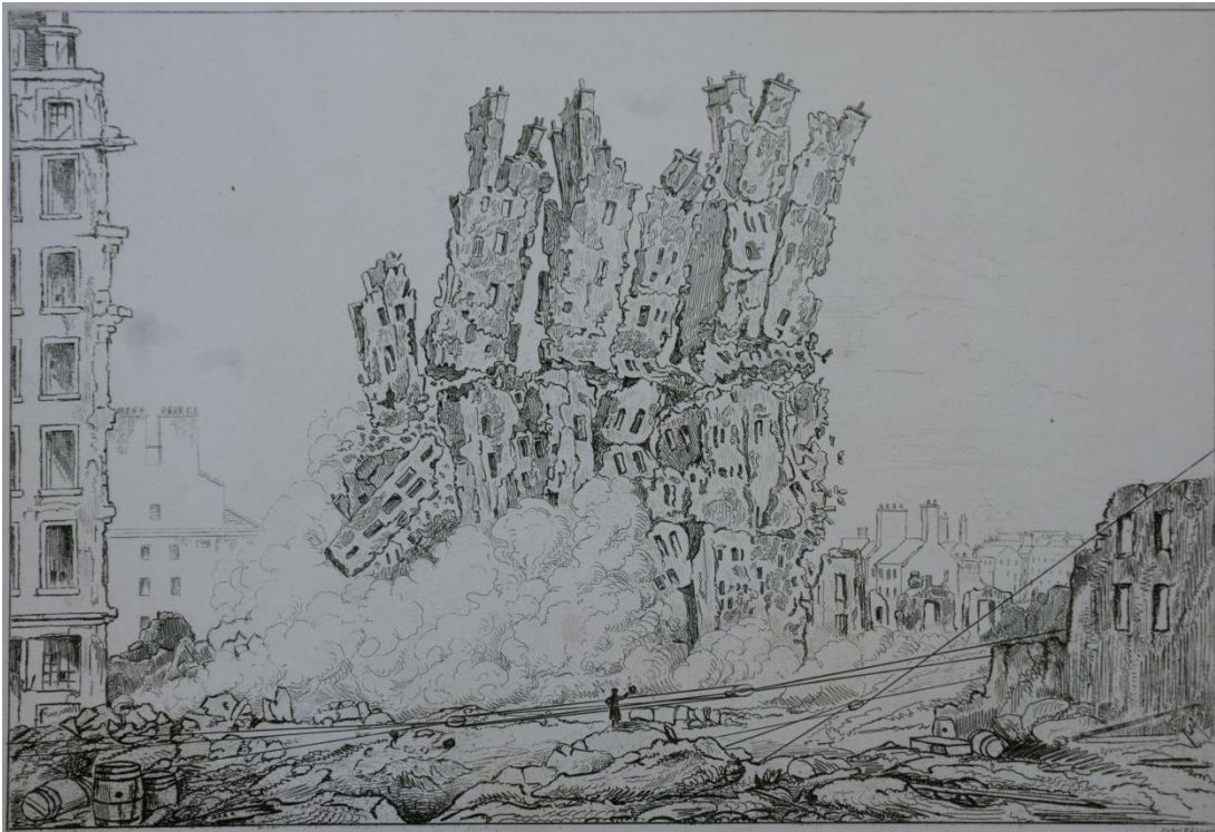
Figure 5.7: Appearance of the ruins on the eastern side of Parliament square the instant after mines were sprung.
