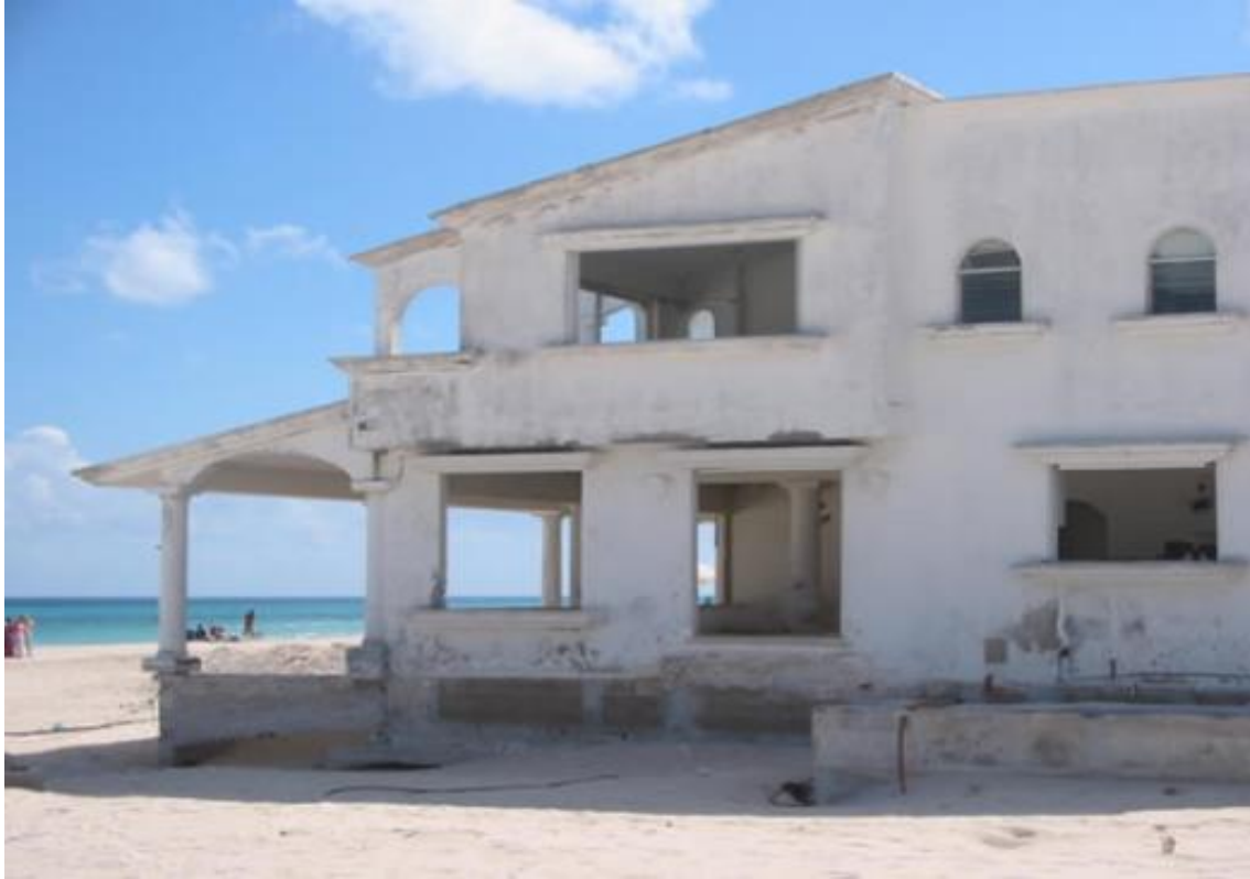
Figure 2-16. An abandoned beach house awaits demolition. Resource: Flickr user Swirlspace
