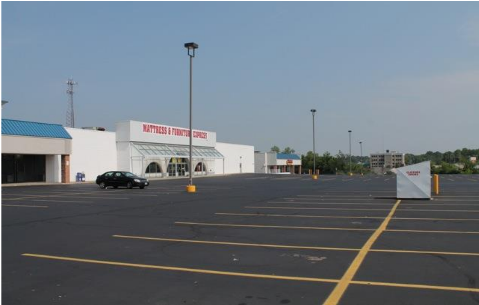
Figure 4-11. Partial View of Main Shopping Plaza Superstructure (Photo courtesy of Rebecca Nocheck)
