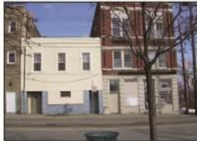
Building exterior lacks address numerics and proper signage.
