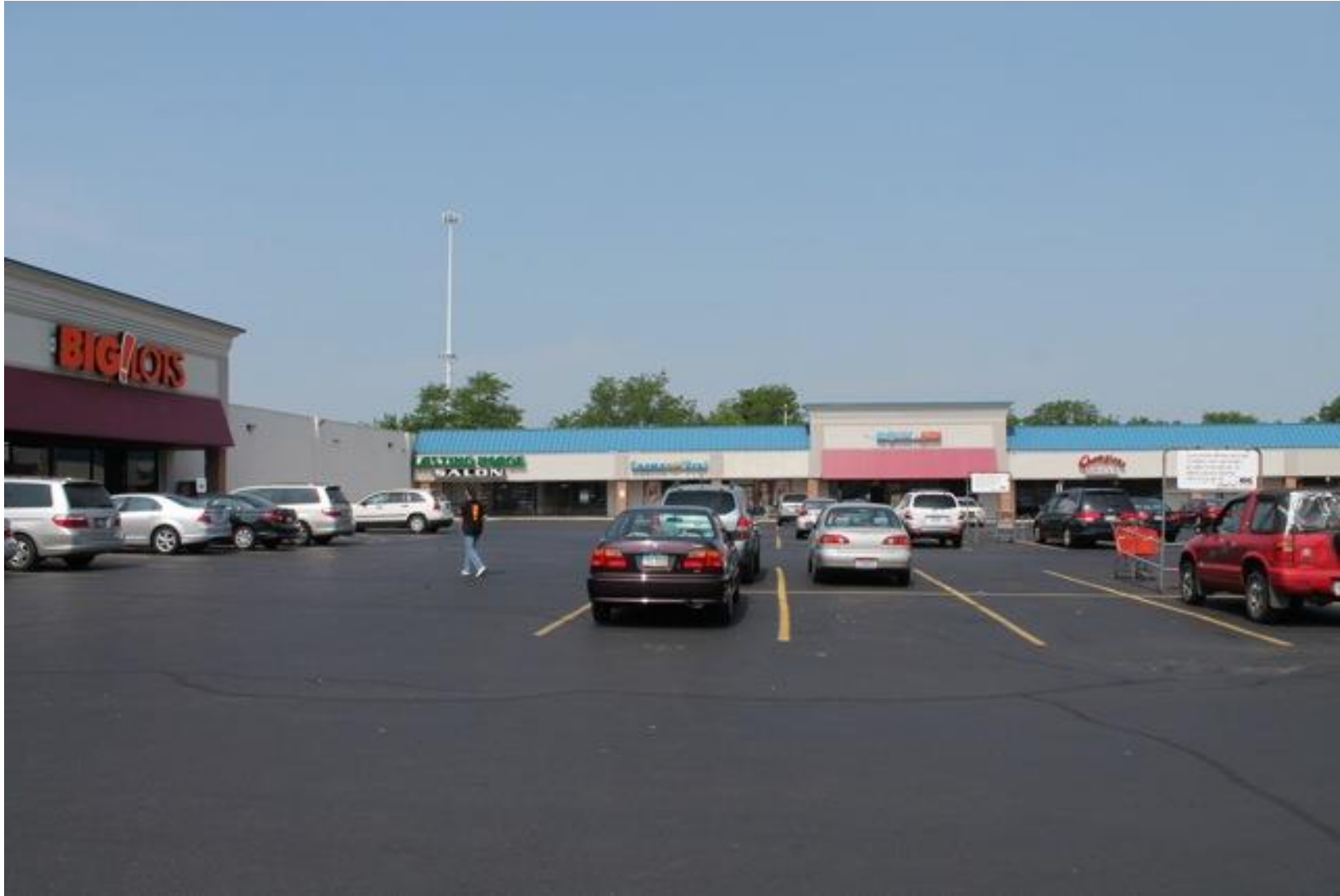
Figure 4-9. Partial View of Main Shopping Plaza Superstructure (Photo courtesy of Rebecca Nocheck)
