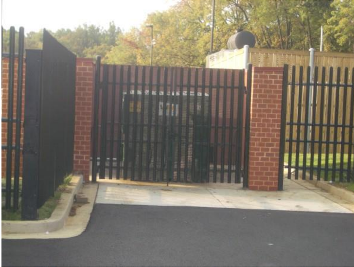
Figure 5-14. Example of properly enclosed dumpster
