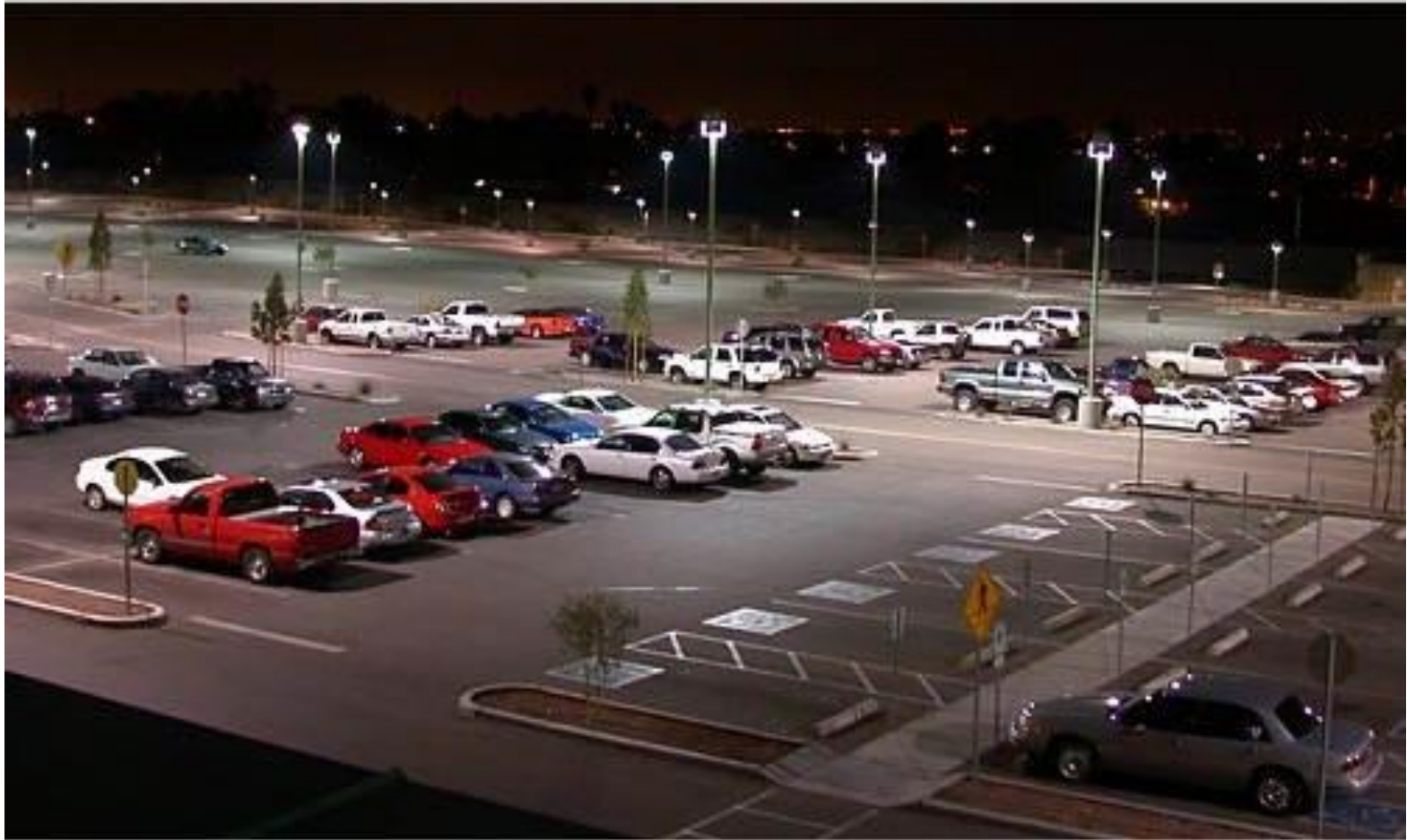
Figure 5-7. Example of a well-lit parking lot (Source: http://www.eltam-eh.com/Parking-Lot_lighting.html )
