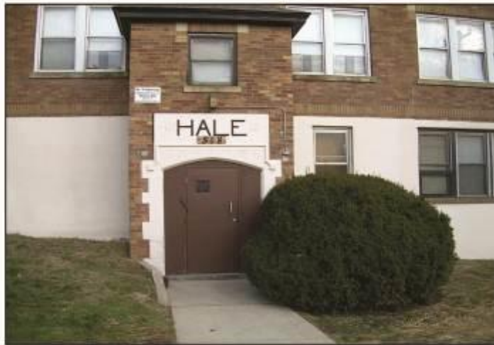
Landscaping is well-maintained, however, foliage provides concealment for criminal element. Property owners should avoid placement of large shrubbery near windows and doorways.
