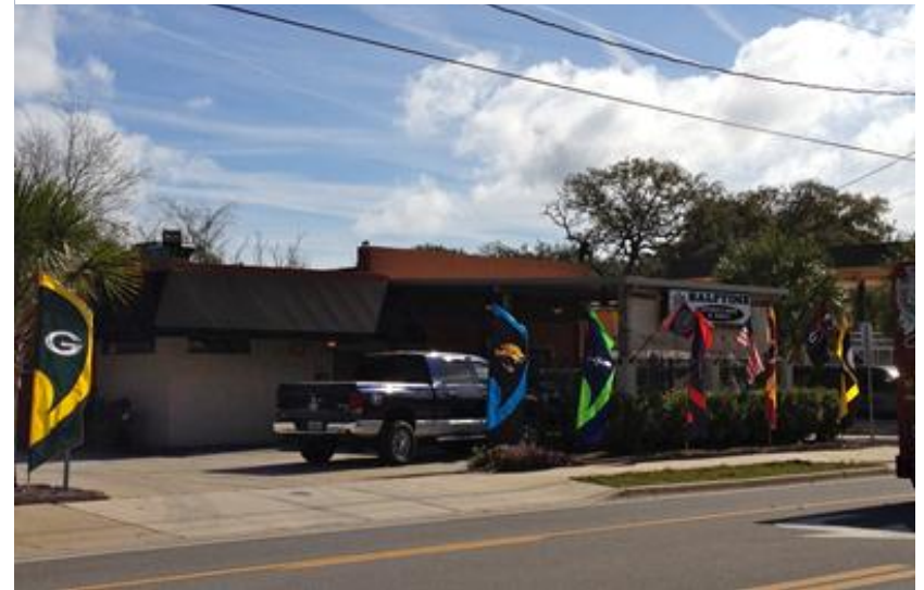
Figure A-24. Gas Station Adaptive Use Examples on 8 th Street
