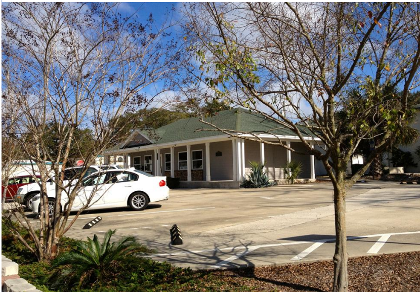
Figure A-23. Gas Station Adaptive Use Examples on 8 th Street
