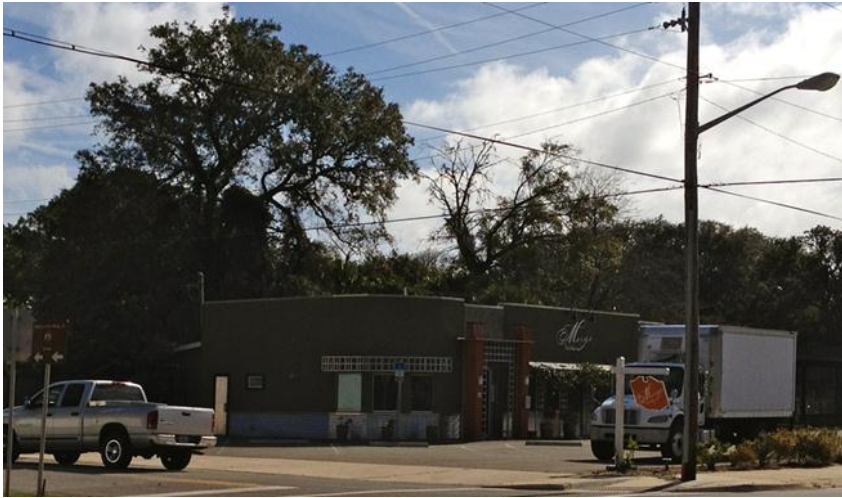
Figure A-21. Gas Station Adaptive Use Examples on 8 th Street
