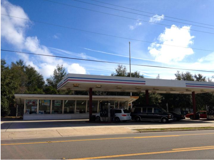
Figure A-8. A1A Gas Station- built in 1962.
