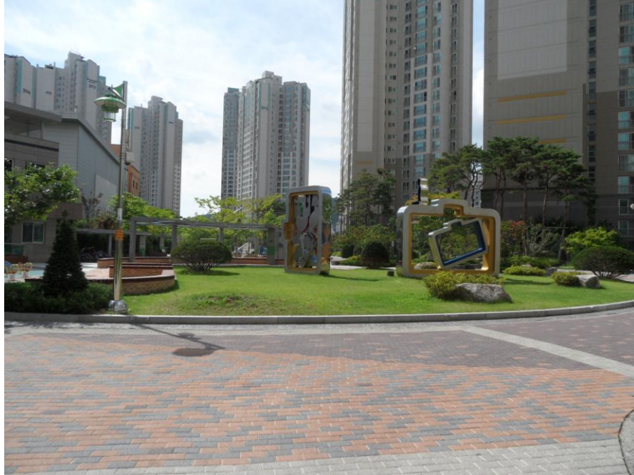
Figure 4-22. Sculptures are located throughout the complex to provide warm and friendly atmosphere. Photograph by author.
