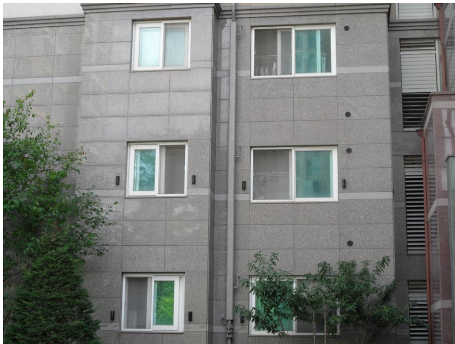
Figure 4-26. Gas pipes covered with specially designed covers to prevent burglars from climbing up. Photograph by author.
