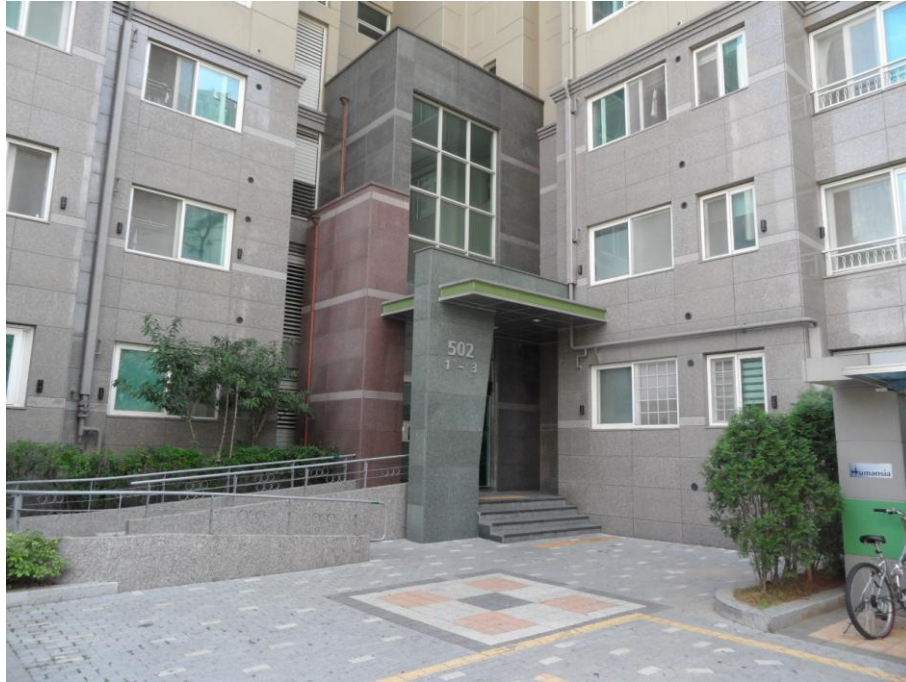
Figure 4-16. Location of the main entrance of the apartment building allows for good surveillance from windows. Photograph by author.
