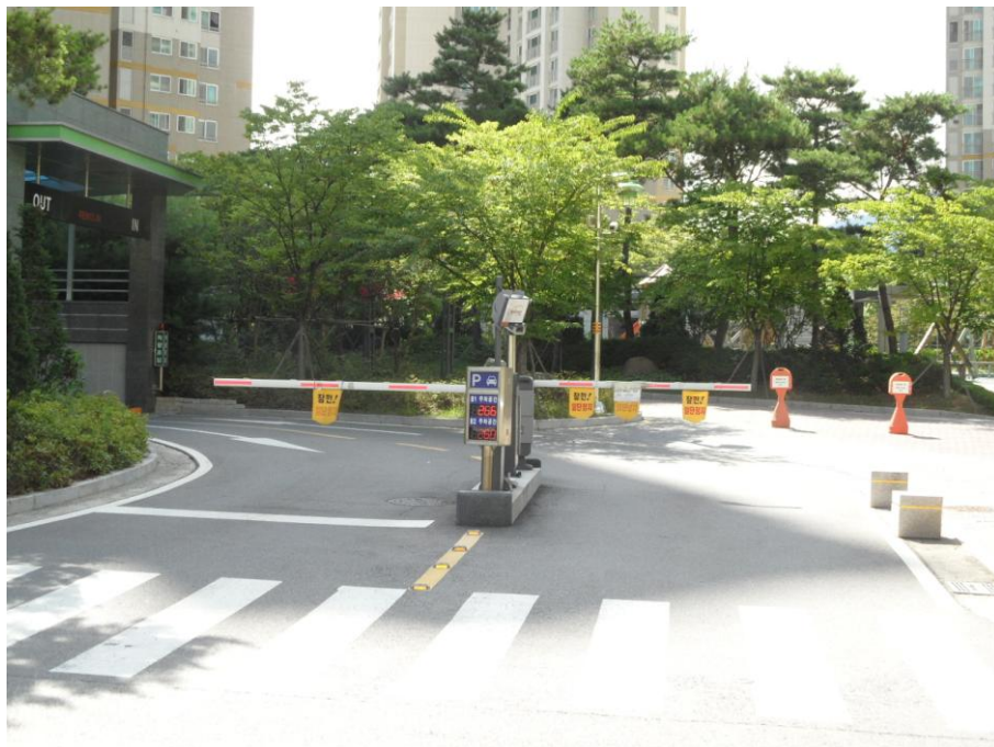
Figure 4-5. Gated entrance. Photograph by author.
