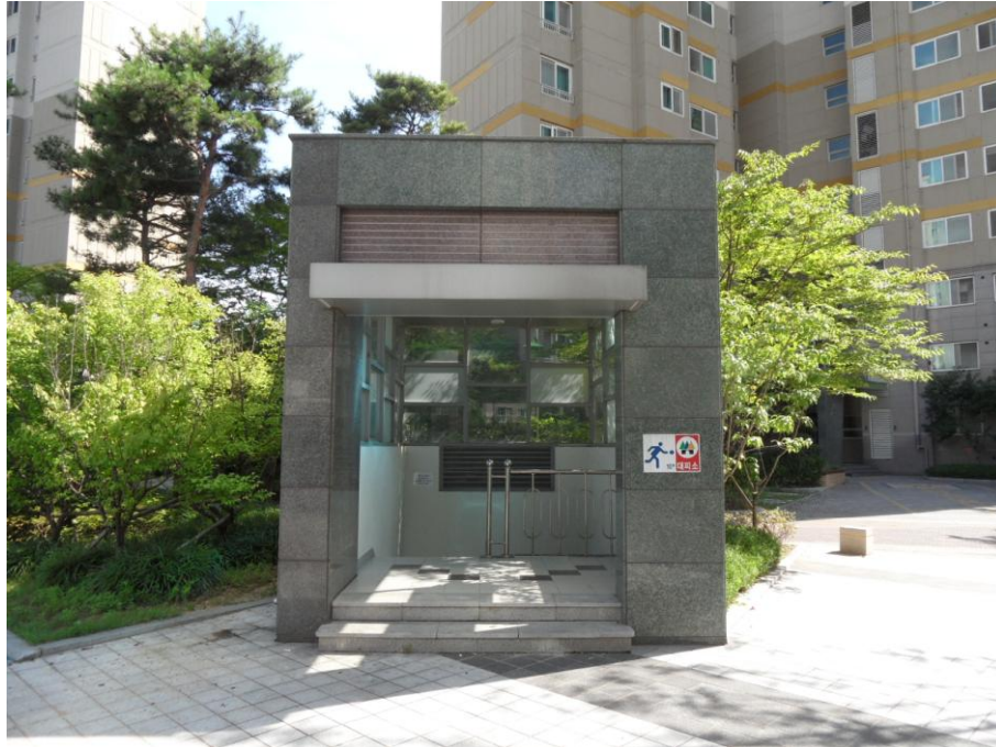
Figure 4-24. Entrance of emergency safety shelter. Photograph by author.
