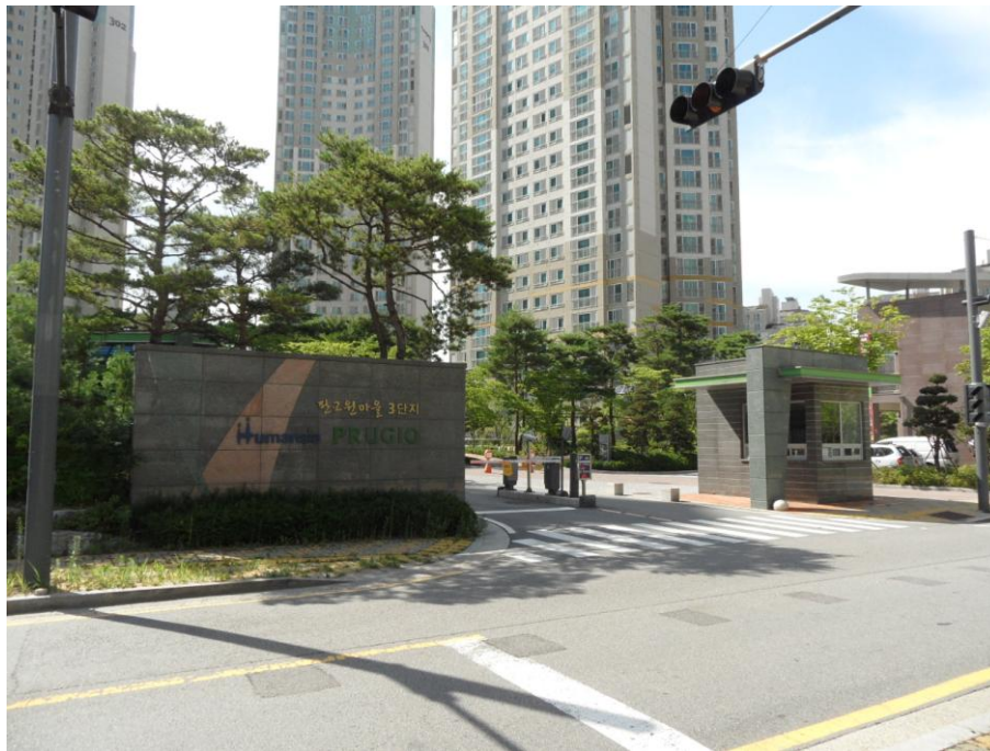
Figure 4-3. View of the main entrance to Pangyo-won Village Community No.3 and No.5 “Humansia-Prugio” with emblem. Photograph by author.
