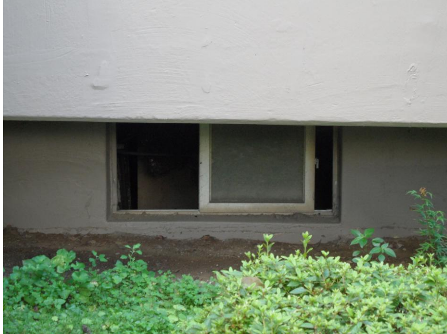
Figure 4-34. Window of the basement of apartment building. Photograph by author.
