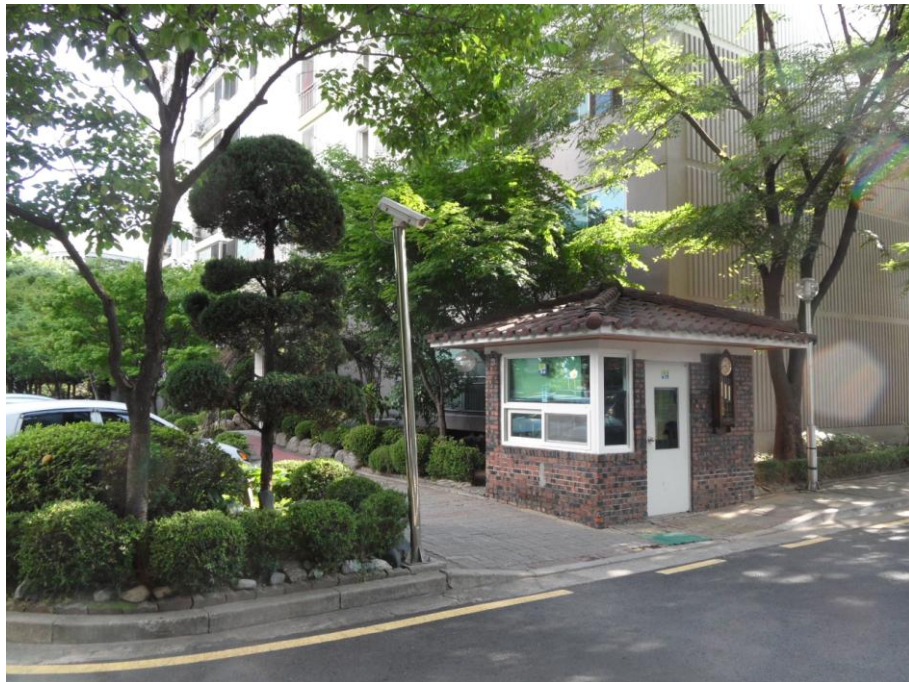
Figure 4-35. Security janitor's office, CCTV camera, and street lamp. Photograph by author.
