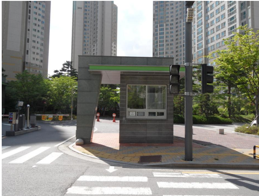
Figure 4-4. Security janitor's office at the entrance. Photograph by author.
