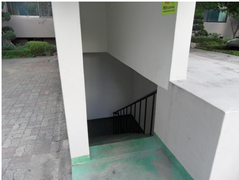
Figure 4-43. Staircase to underground parking lot. Photograph by author.
