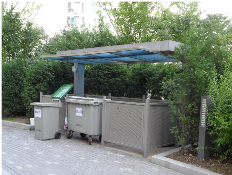
Figure 4-25. Waste disposal located under a shelter with lighting system installed beside. Photograph by author.
