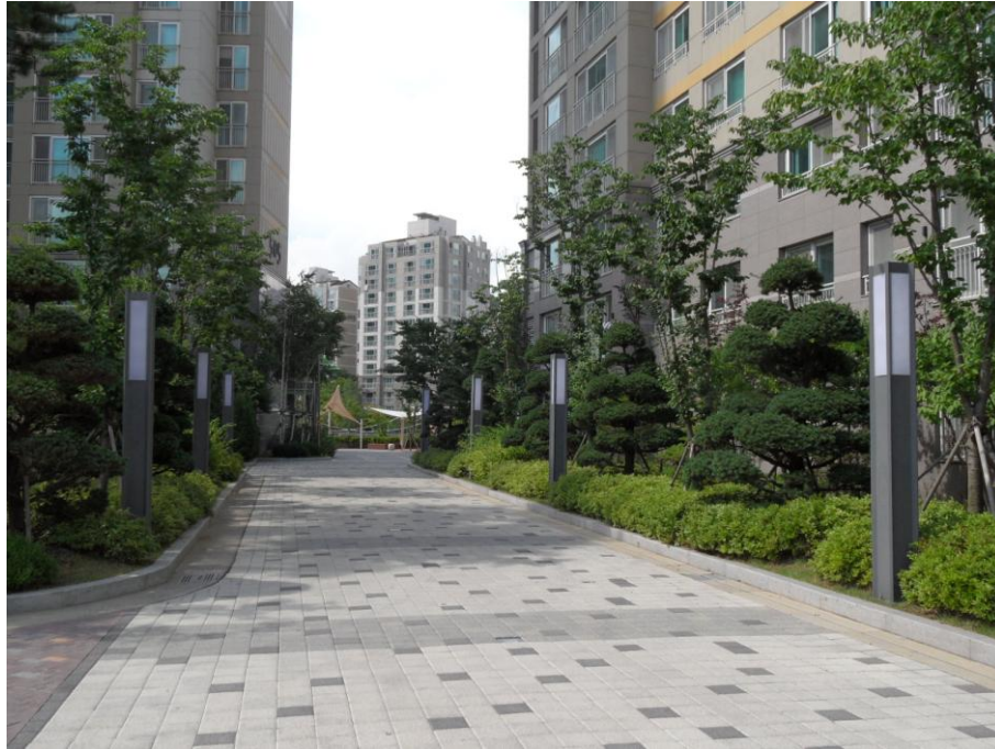
Figure 4-14. Designed lighting systems installed along the pavement. Photograph by author.
