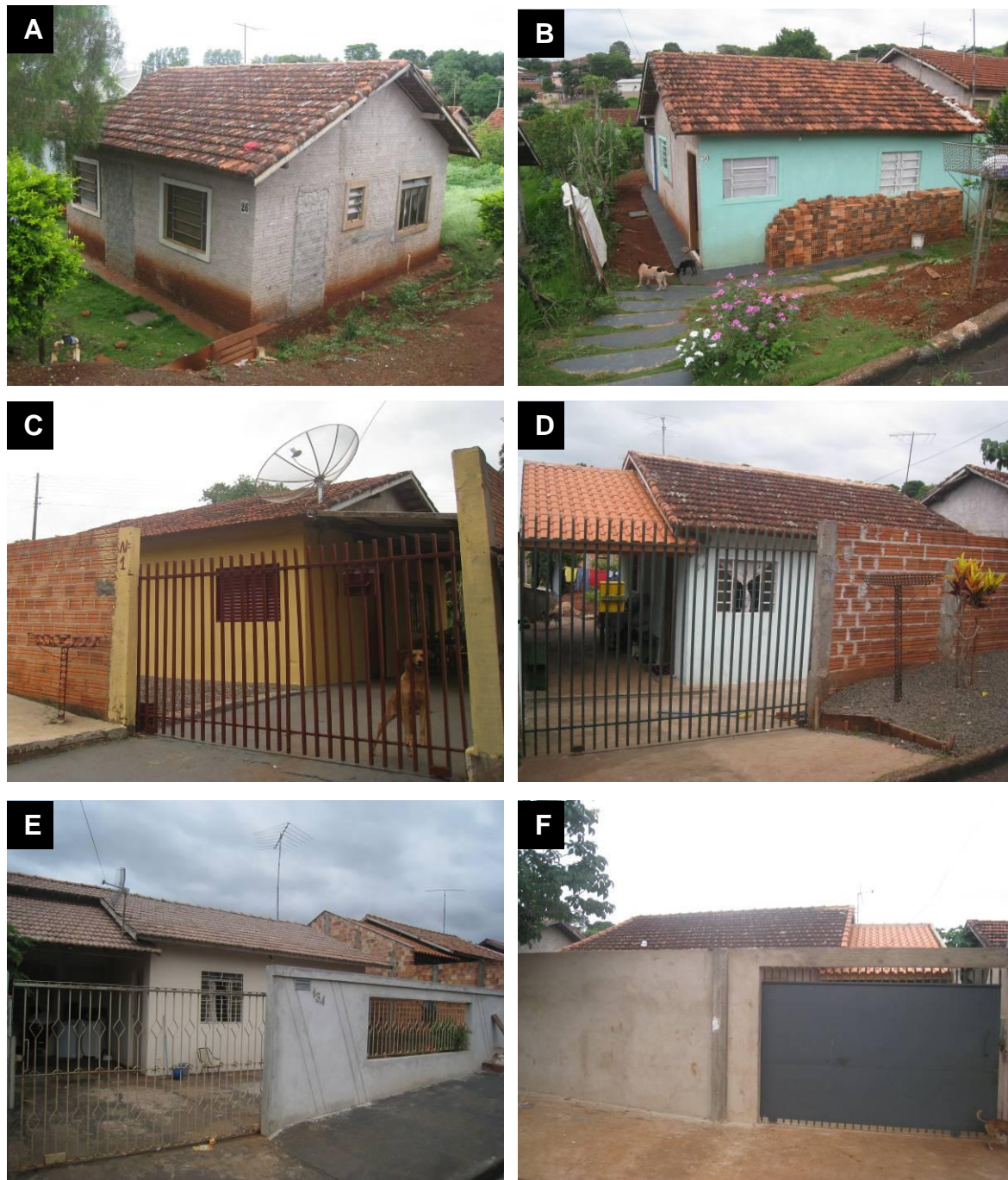
Figure 5-5. Improvements in the houses of 'Hope Village'. A) House with front door transferred to the side, B) house that has been painted and had the windows replaced, C) house that has been painted, fenced and expanded, E) and F) units that have undergone radical change in comparison to the original design. Source: Pictures by author.
