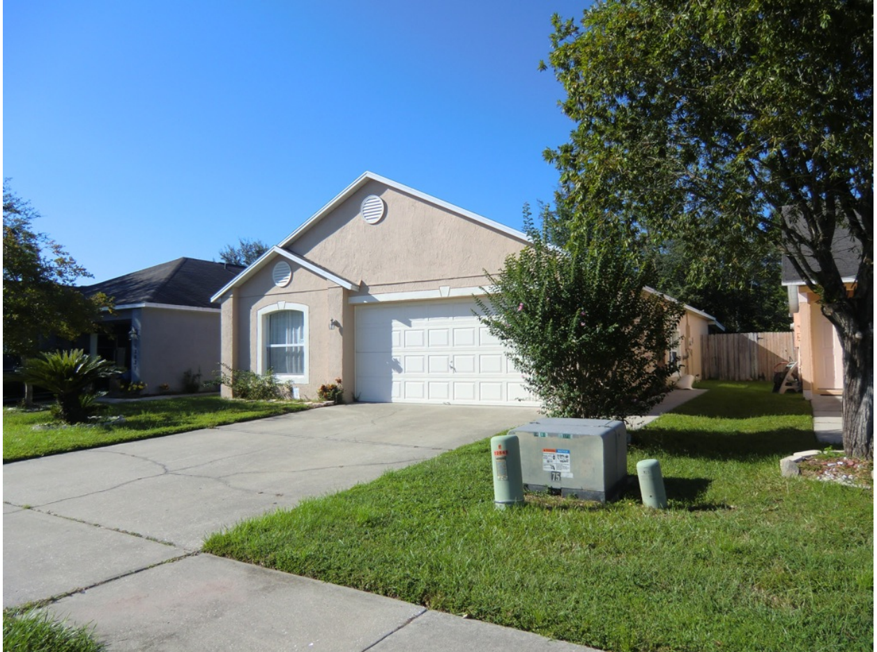
Figure 4-16. Dispersed and exposed parking. Some homes do not have a front door, but have a façade dominated by a garage door.
