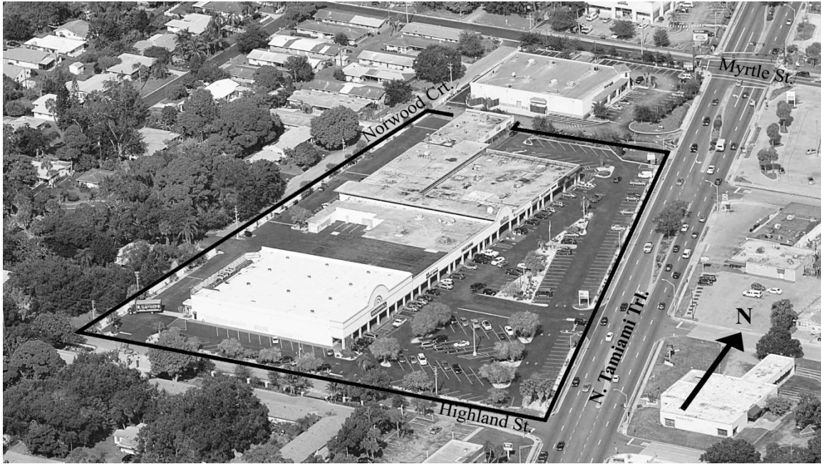
Figure 3-17. Trail Plaza aerial view, facing northwest. Source: Greenberg, 2011
