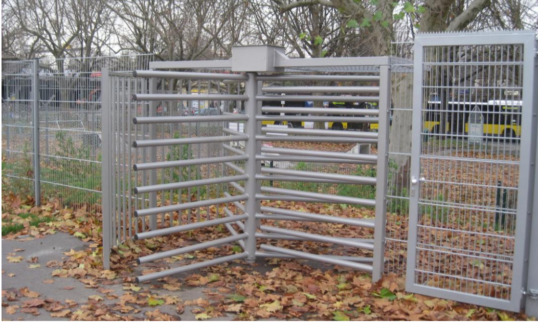
Figure 4-7. Exit gate installed in the fence at Templehof Park. Photo courtesy of James Beeler
