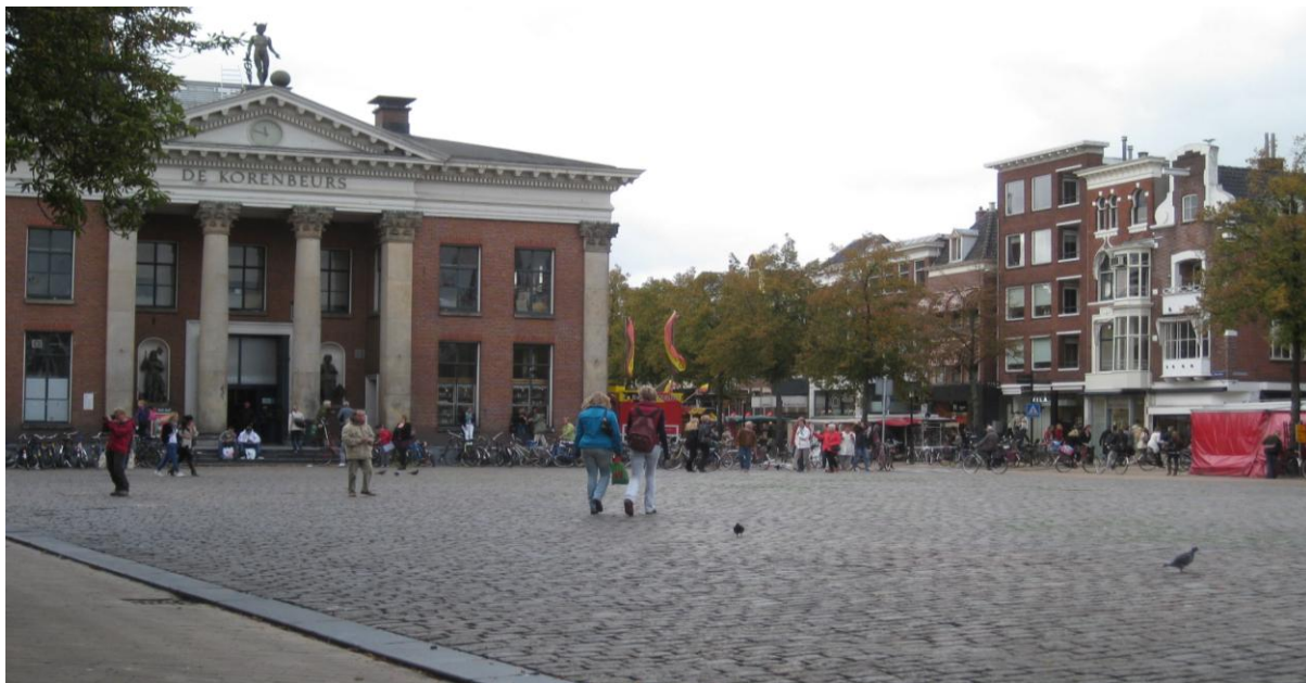
Figure 1-8. Groningen, The Netherlands. Old market hall facing the fish market square. This building is now a modern food market. Photo courtesy James Beeler.
