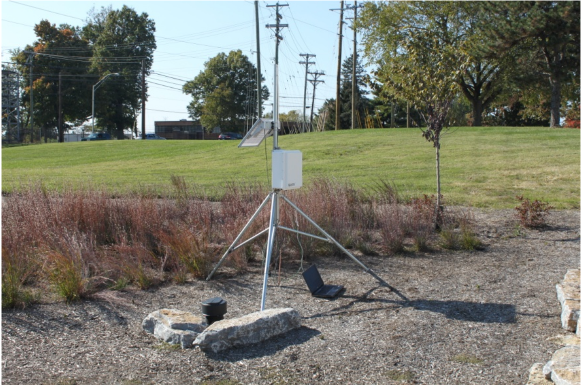
Figure 3.9. An EnviroScan soil moisture sensor with a Campbell Scientific datalogger (shown) were used to collect soil moisture data at seven vertical intervals.
