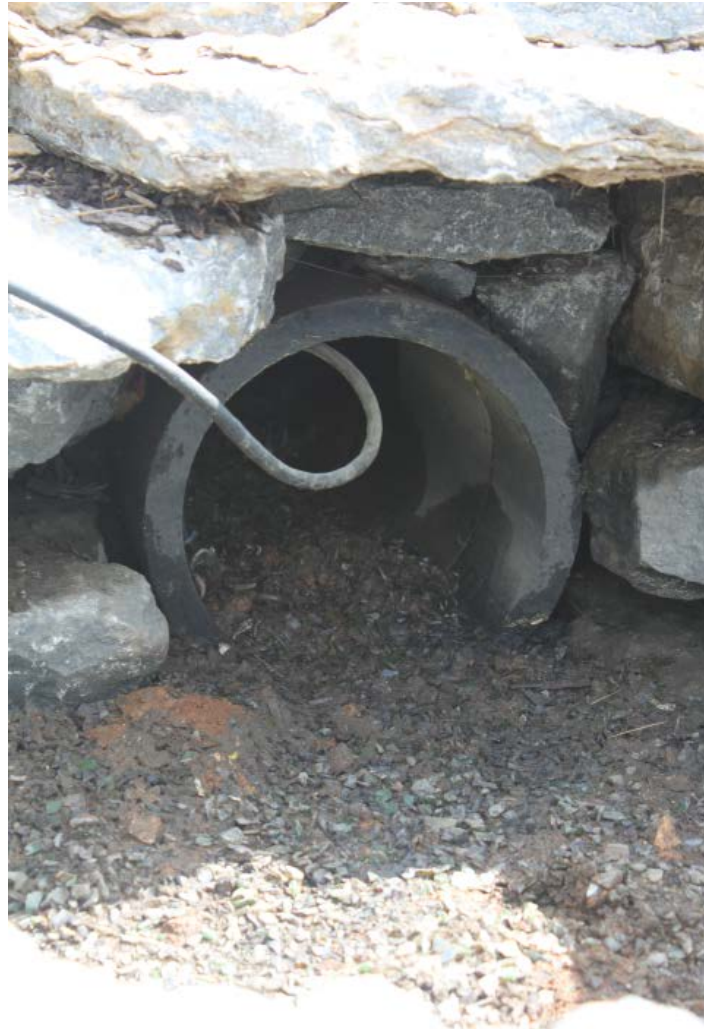
Figure 3.8. Sediment placed in the 30 cm HDPE pipe by a groundhog.
