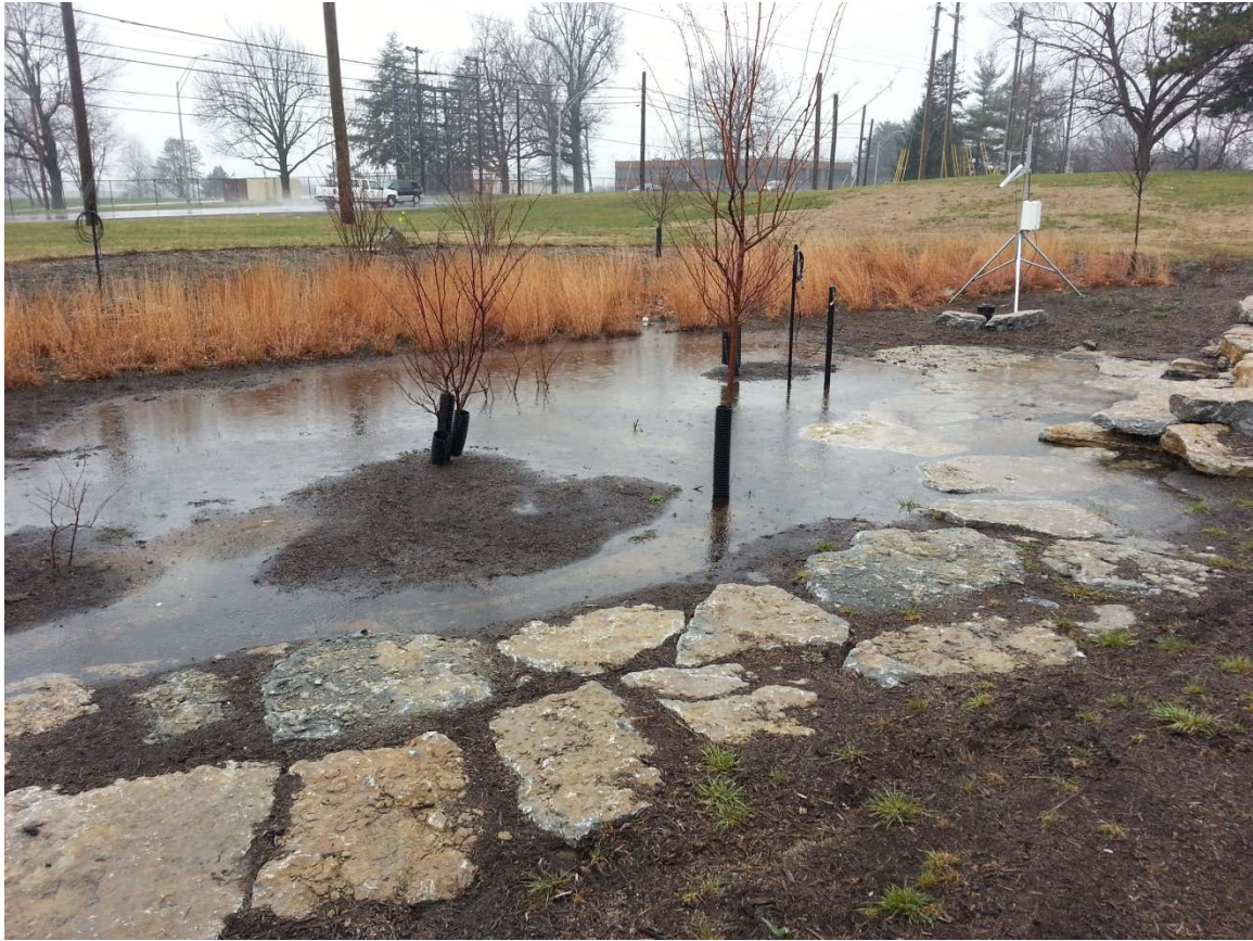
Figure 3.11. Ponded water was observed in the rain garden on March 24, 2013.
