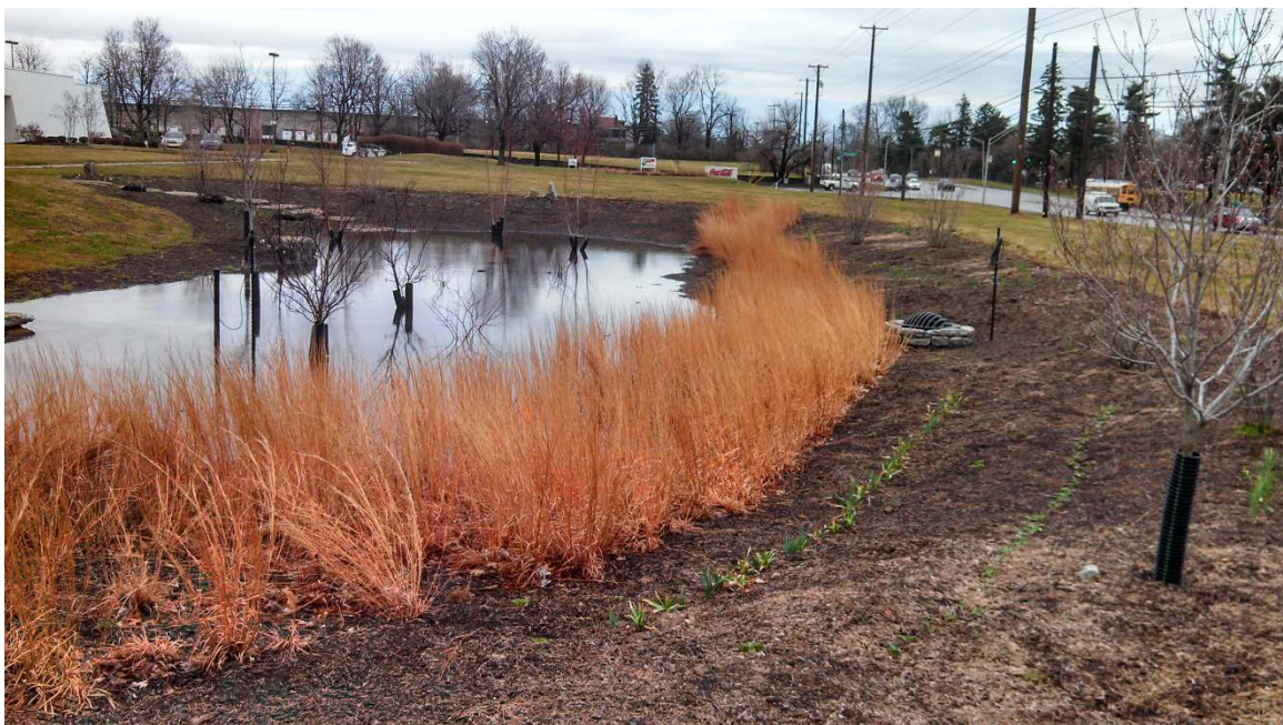
Figure 3.12. Ponded water was observed in the rain garden on March 18, 2013.
