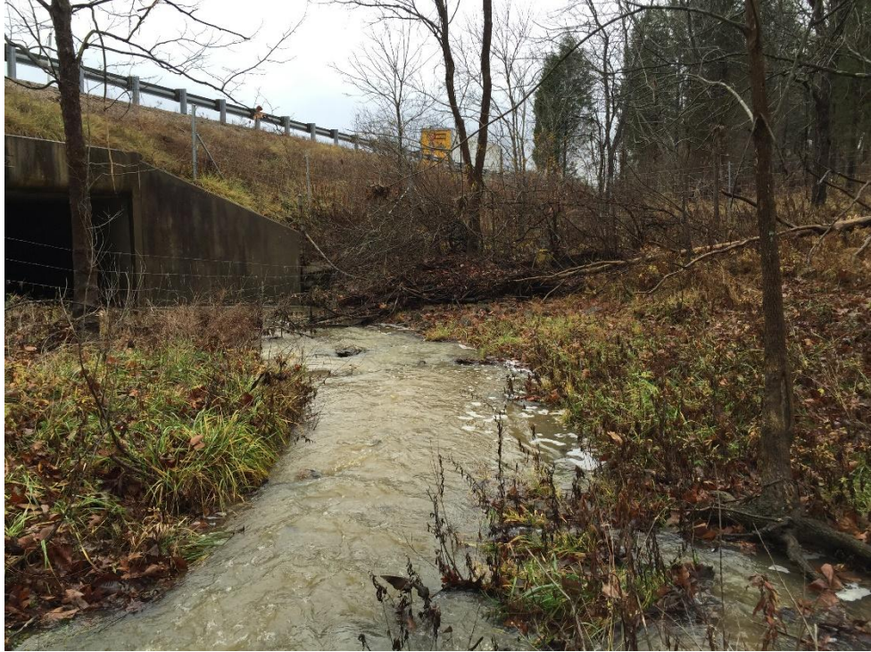
Figure A.4: Downstream view of Site ID 3: USGS gage 03250150 Indian Creek (HLR 9).
