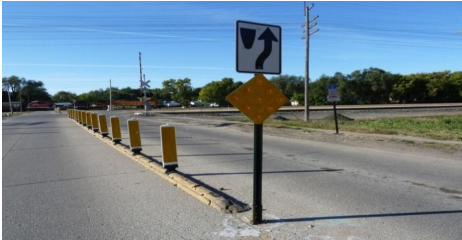
FIGURE 3.3 Barrier condition after maintenance
