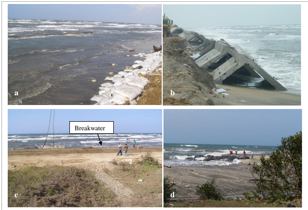
Figure 5. Shore protection measures installed at the 20 th km. a,b,c. Breakwater made with panels of reinforced concrete (Photos taken in April, 2011 by author). d Sandbags installed to trap sediment (Photo taken from the road toward the northeast on May 28 th , 2014 by Cristóbal Pizarro).
