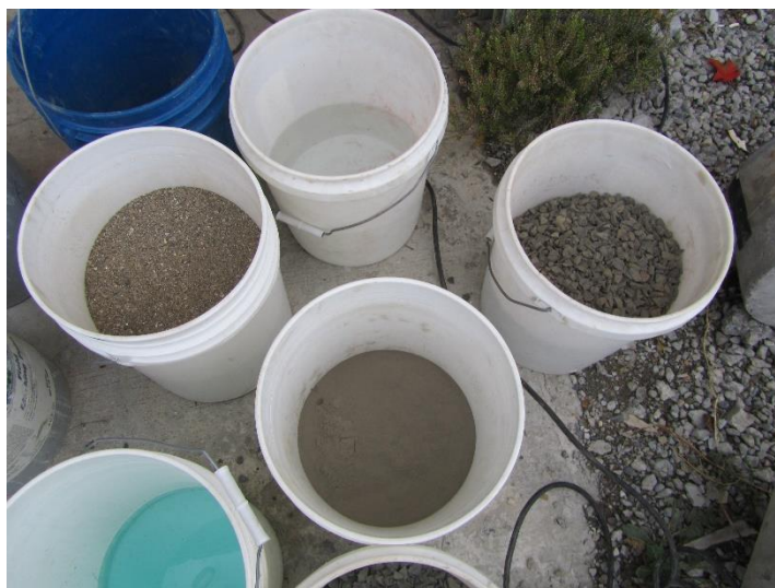
Figure 4-1: Measured Concrete Constituents Before Mixing
