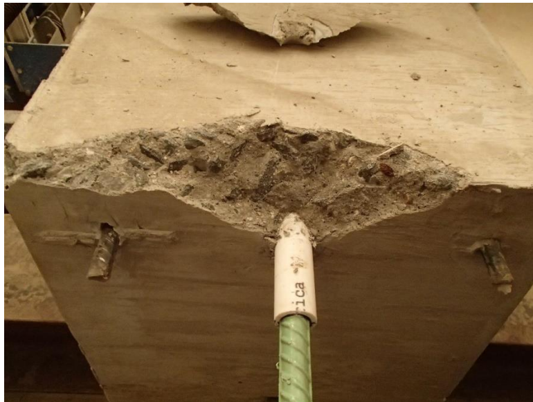
Figure 5-12: Concrete Cracking in Bar Pullout Tests with No.4 Test Bar
