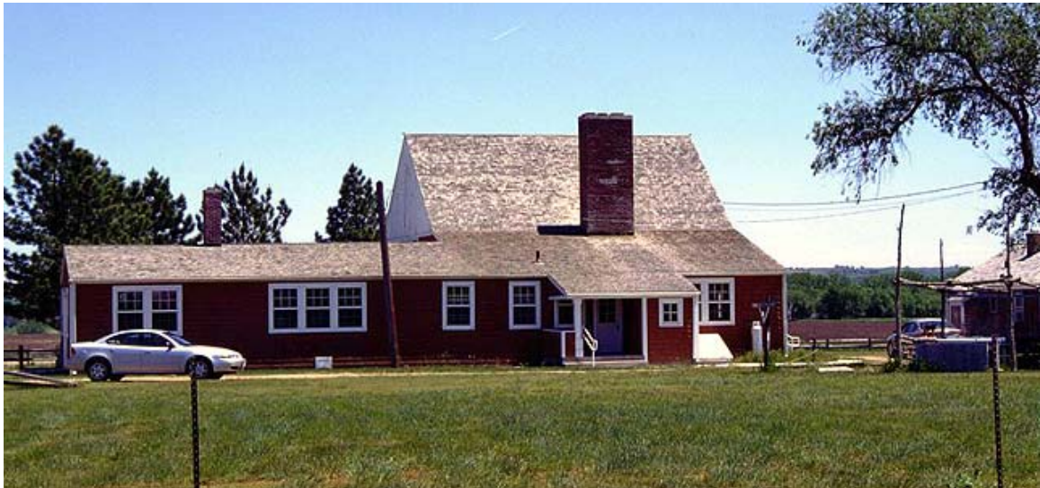
Figure 4.13, Ponca Tribal Self-Help Building (Nebraska State Historical Society 2009)
