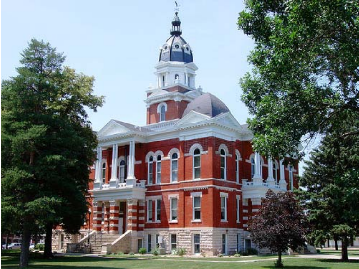
Figure 3.4: the Johnson County Courthouse (Jones 2009)
