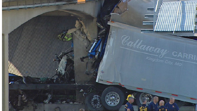
Figure 1.3. Tractor-trailer collision with the I-30 bridge over Dolphin Road (Vega 2012)
