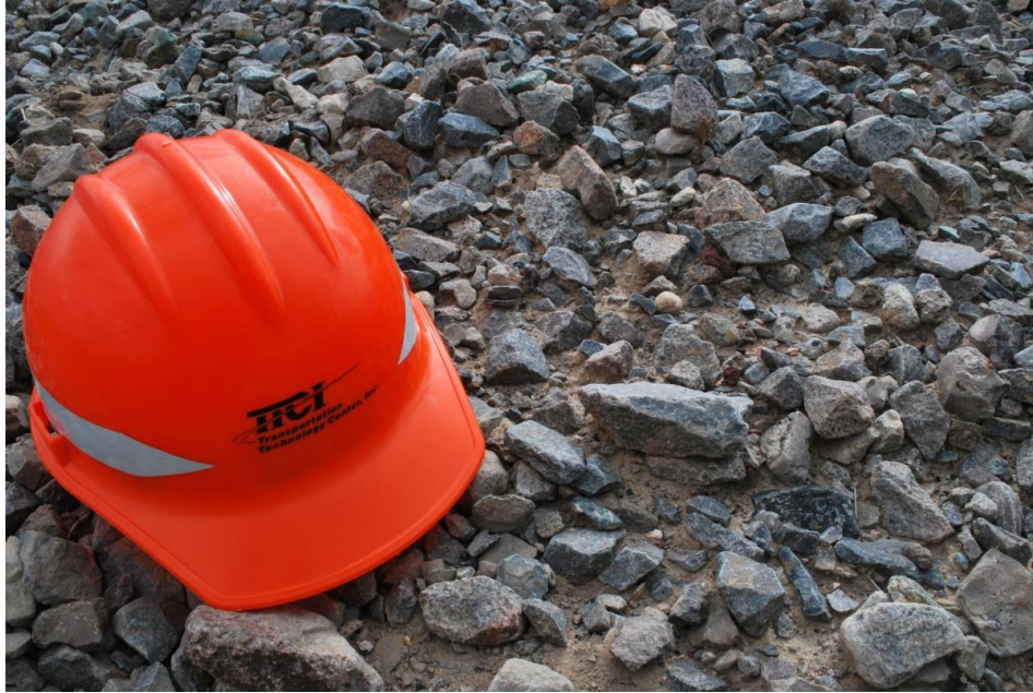
Figure 1.3 An example of fouled ballast
