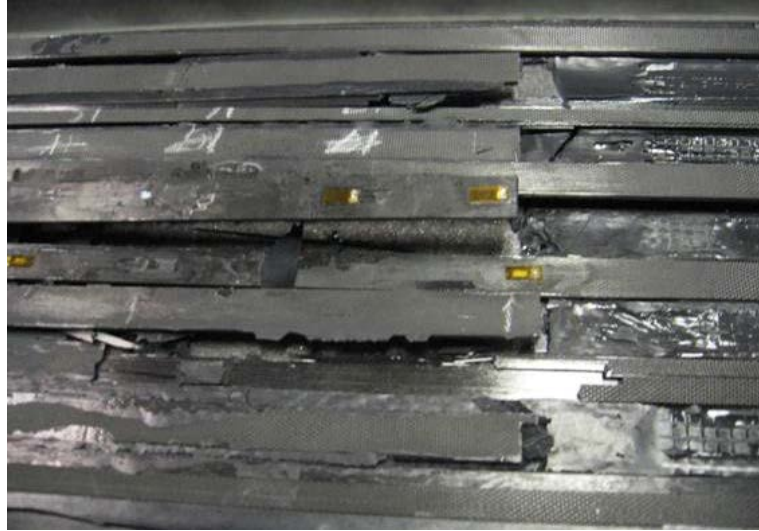
Fig. 2.45: Debonding at mid span ‘finger’ joint
