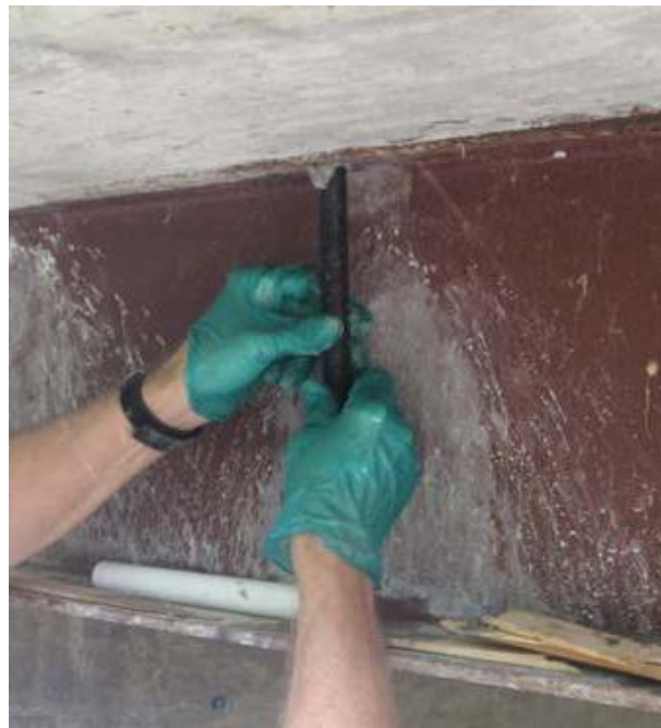
Fig. 5.10: Inserting threaded rod with twisting motion
