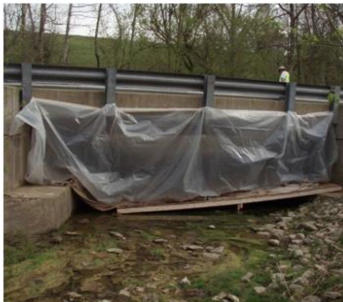
Fig. 5.13: Temporary platform and enclosing for grit blasting
