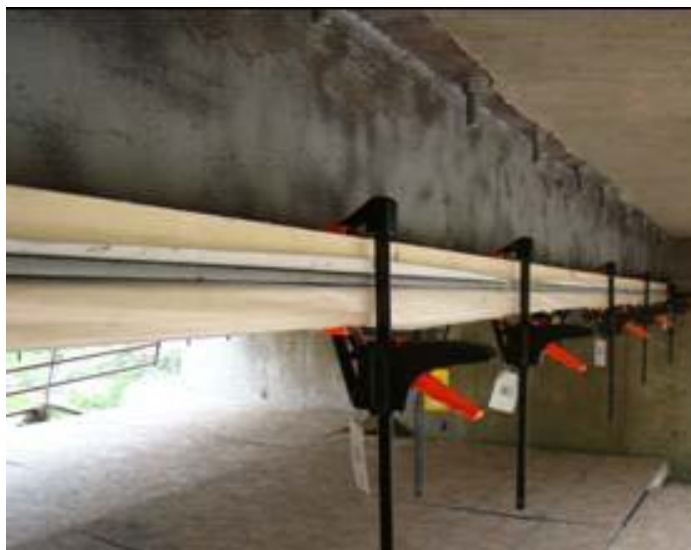
Fig. 5.21: Clamping both top and bottom laminates
