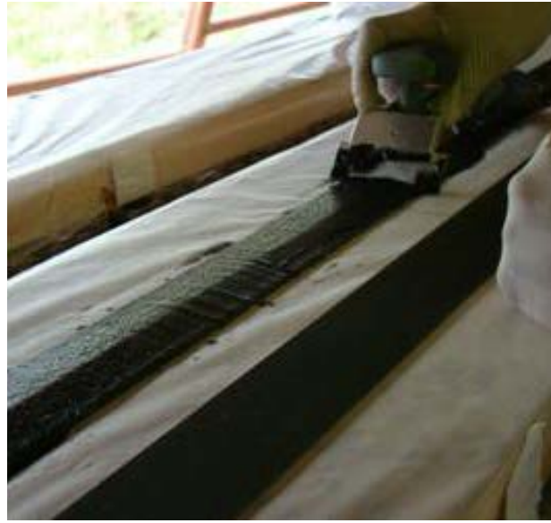
Fig. 5.19: Spreading of epoxy with V-notch trowel
