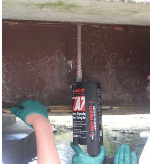
Fig. 5.9: Inserting of adhesive into drilled hole
