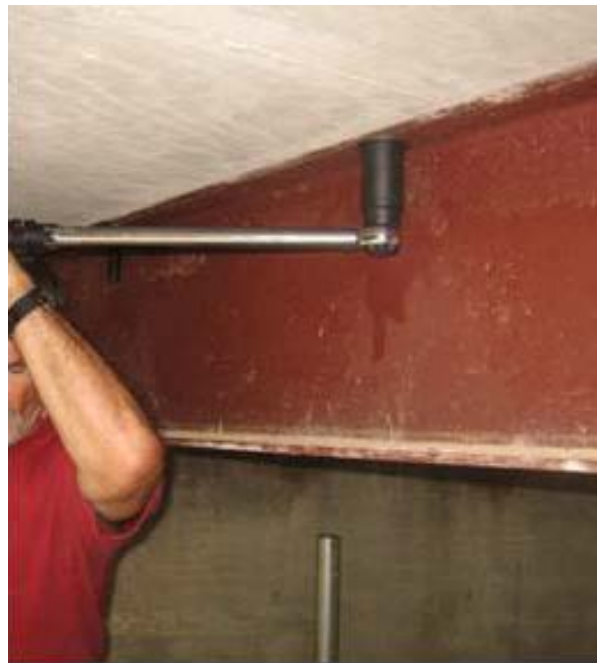
Fig. 5.12: Tightening of nut to specified torque
