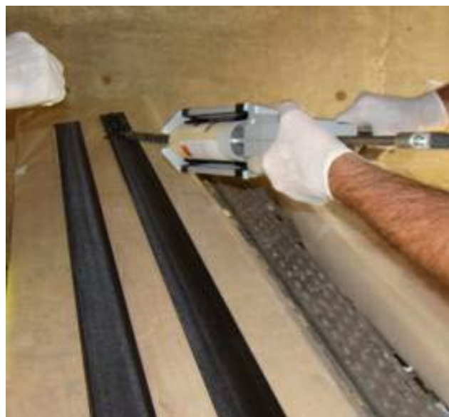
Fig. 5.18: Application of epoxy on to the top surface of the laminate
