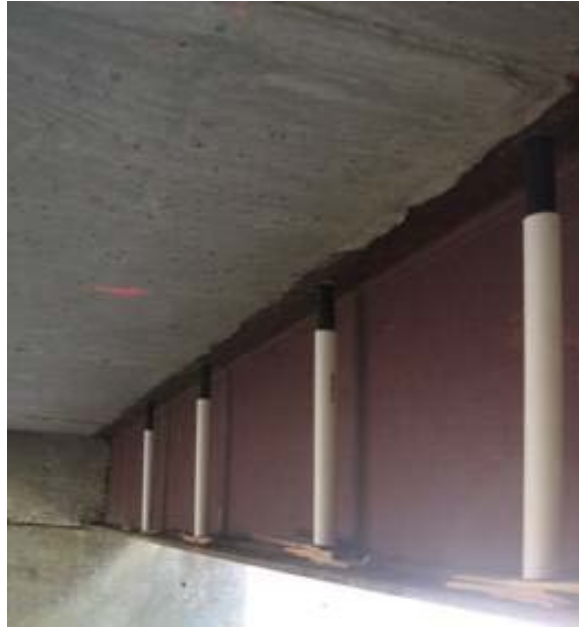
Fig. 5.11: Threaded rods held in place during curing
