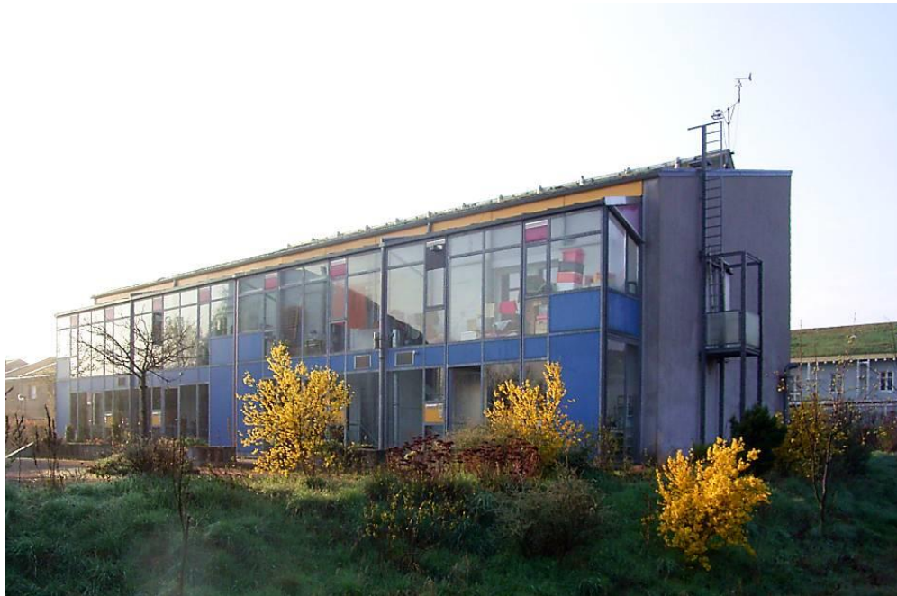
Figure 4.6: View of the North side of the passive house at Darmstadt Kranichstein
