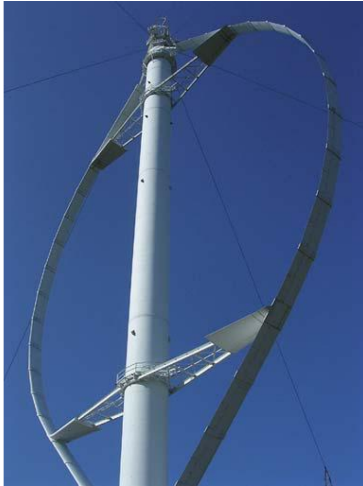
Figure (3-13) A 4.2 MW vertical axis Darrieus wind turbine. (Source: www.reuk.co.uk ).
