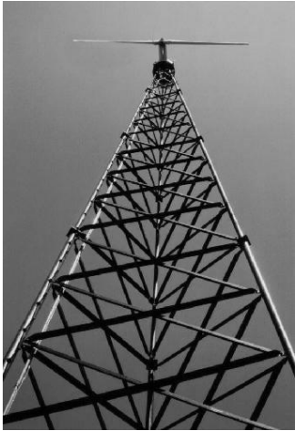
b) Lattice tower
