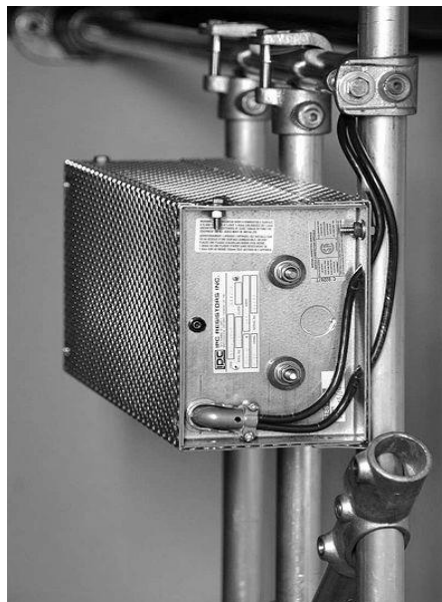
Figure 2.3: Dynamic braking resistor for wind turbine
