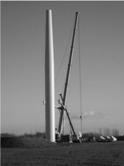
c) Concrete tower
