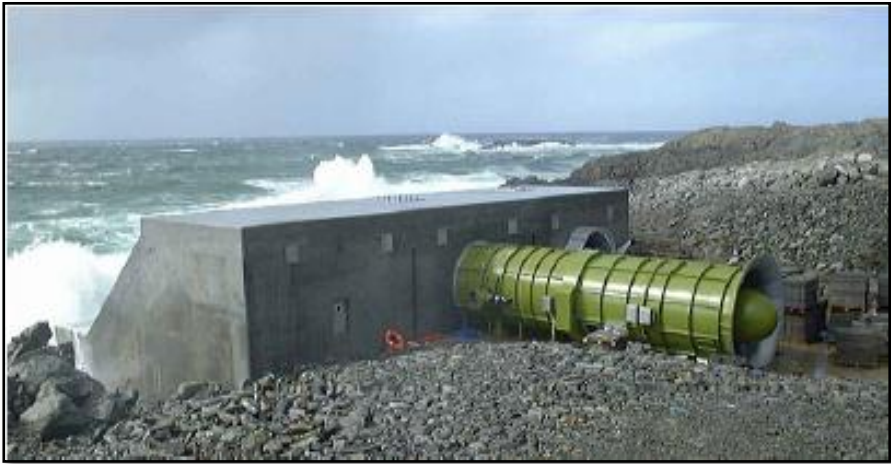
Figure (3.6): The LIMPET project in Islay installation.
