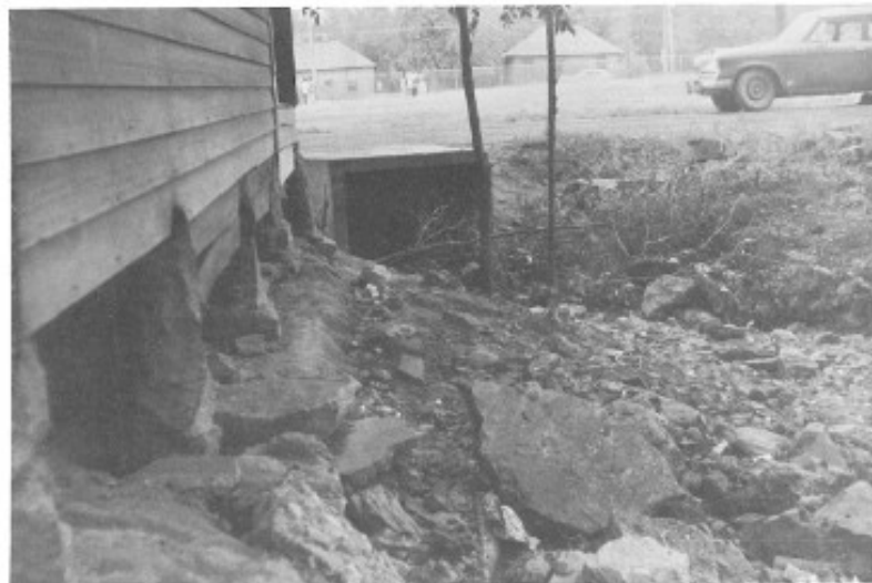
Open ditch west of Fifth Street.
