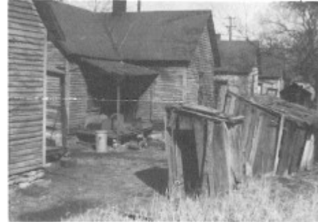
Outside pit toilets.
