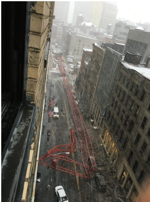
Figure 4: Boom Damage of the Collapsed Crane in Manhattan [3].
