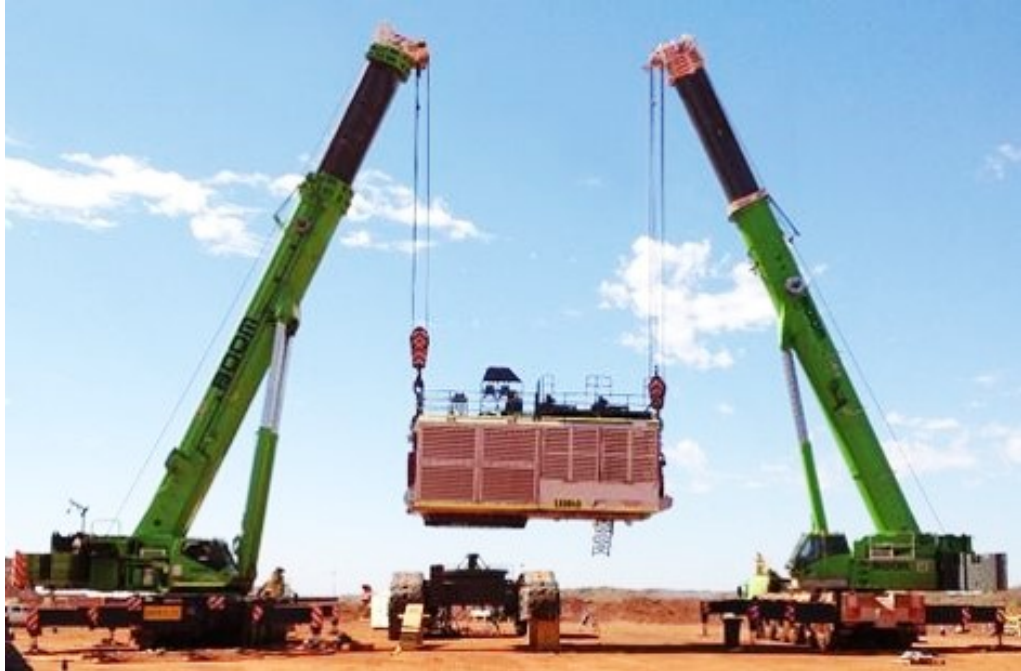
Figure 80: Tandem Lifting Cranes [36].
