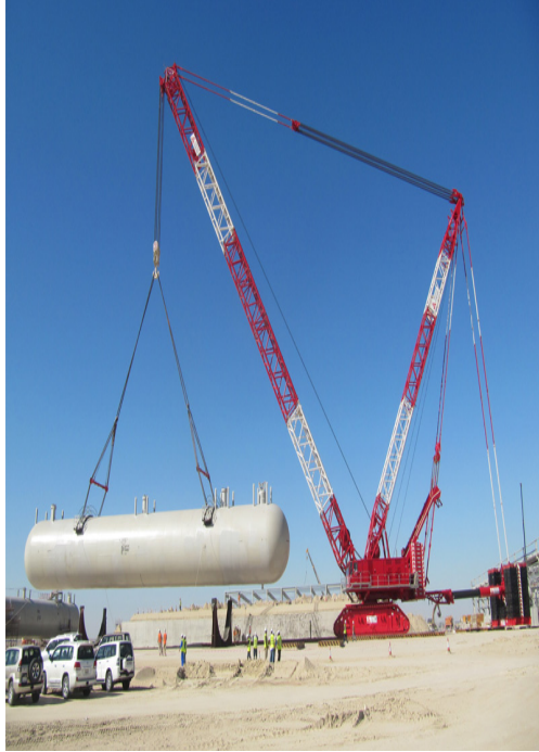
(a) Mobile Crane [21]
