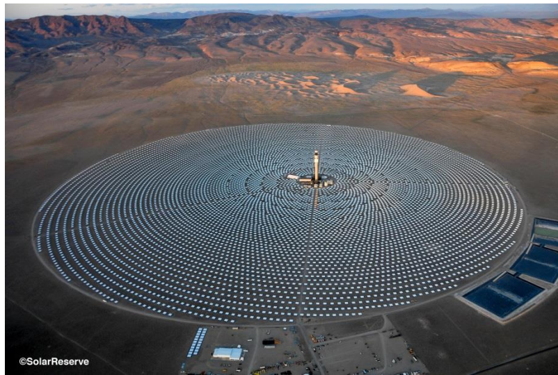
Fig. 4: Crescent dunes LS-CSP plant (Solar Reserve)
