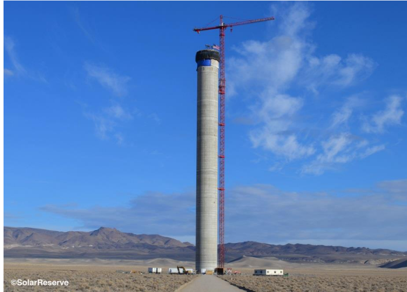
Fig. 9: An example tower constructed for the Crescent Dunes CSP plant in Nevada
