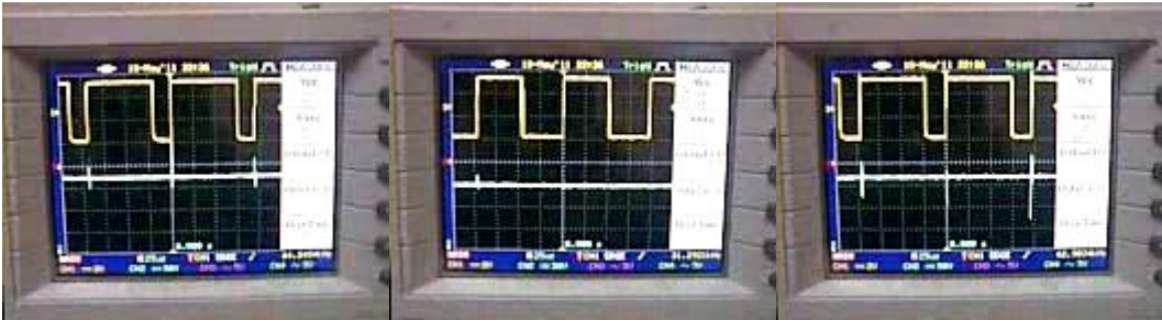
Figure 6-21: Examining the PWM output with open loop controller.
