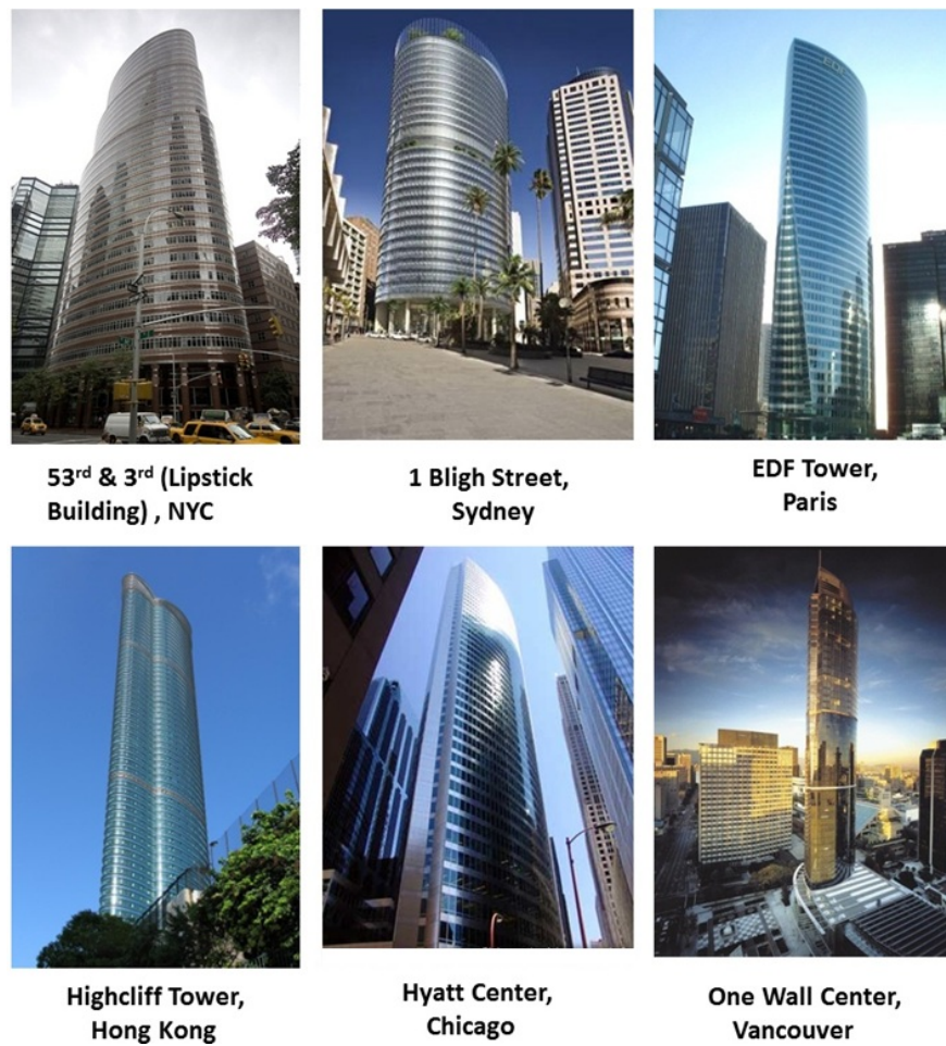
Figure 23: Example of streamlined cross-section high-rise buildings
