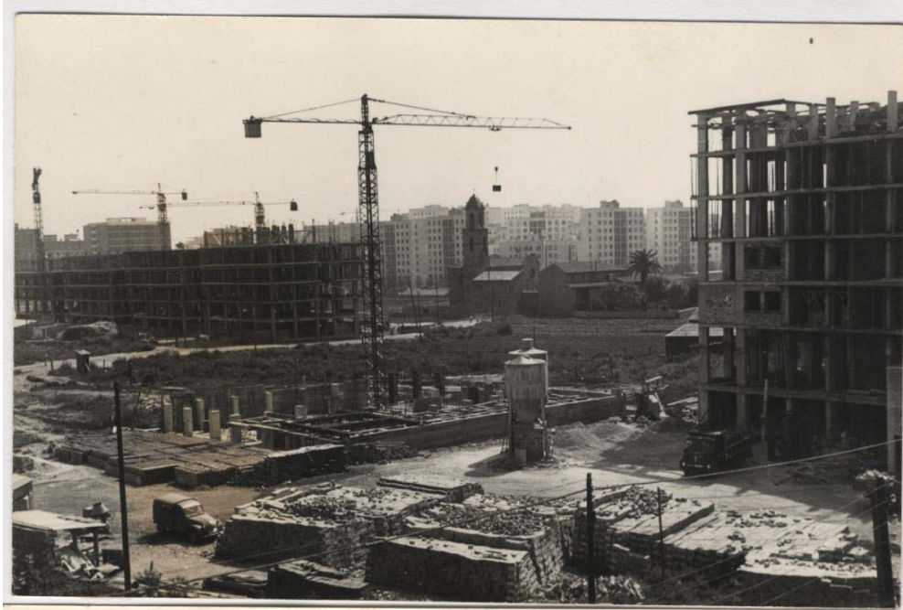
Illustration 18- Construction work in the once crop fields of La Verneda
