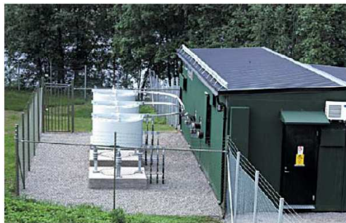
Figure 2.1: Voltage Source Converter Based STATCOM
