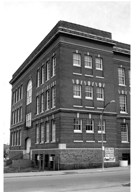
Image C.1 Jackson Elementary School in St. Louis place is closed and the property is up for sale.
