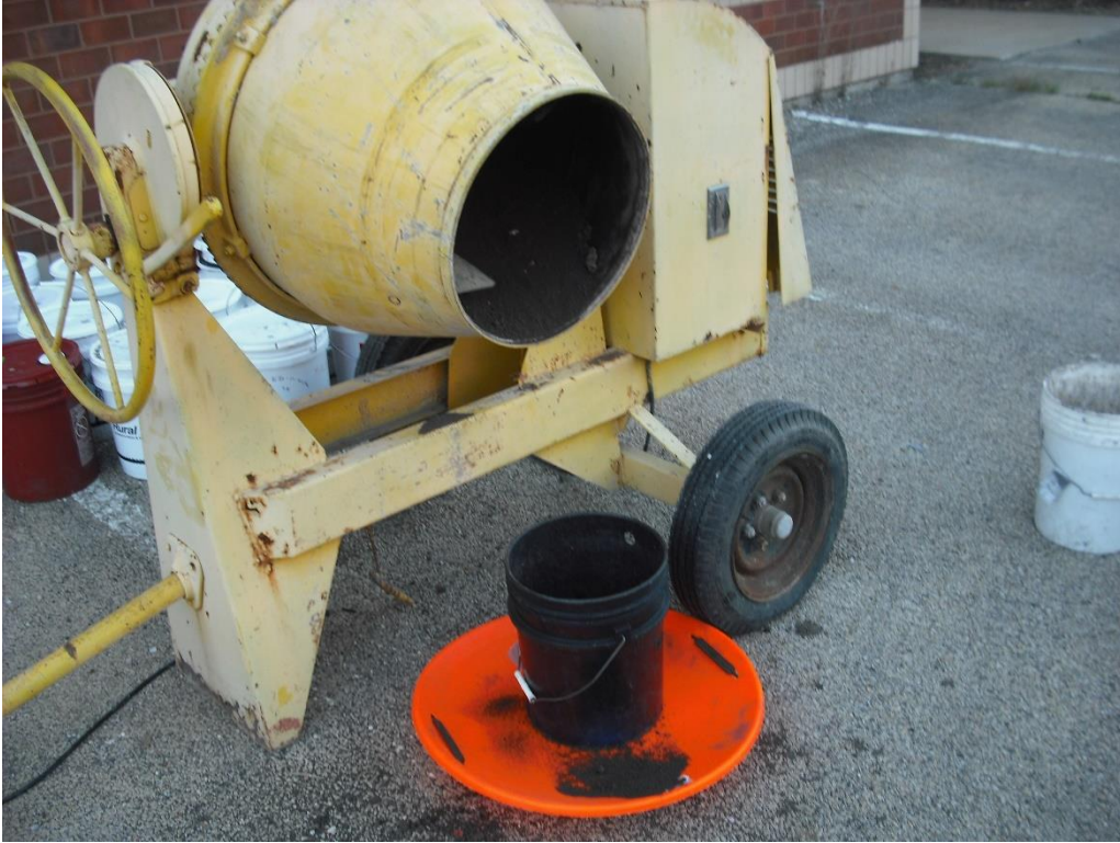
Figure 4.7: Concrete mixer dumping REE mixed soil into bucket
