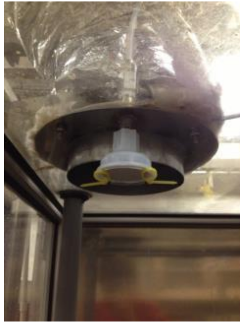
Figure 4.1: Chamber ceiling showing sampling line filter.
