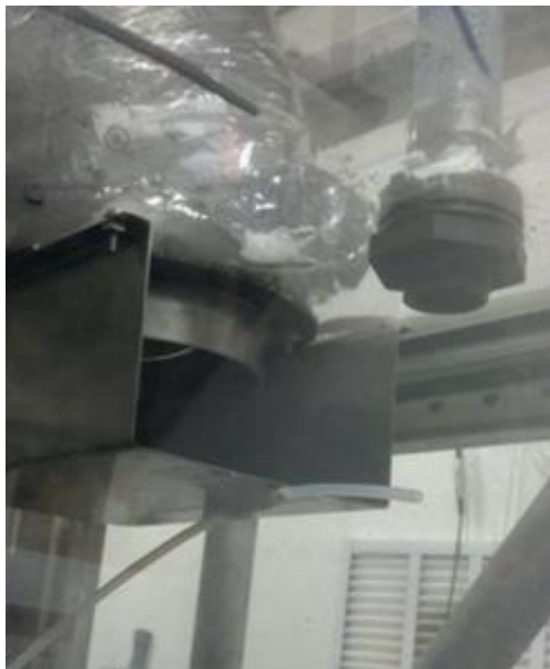
Figure E.2: Injection point taped next to ventilation port.
