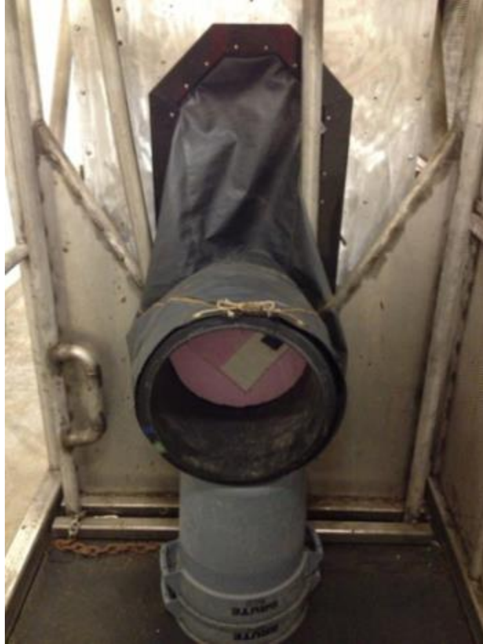
Figure E.1: Hood blocked using Styrofoam board set within plastic tube.
