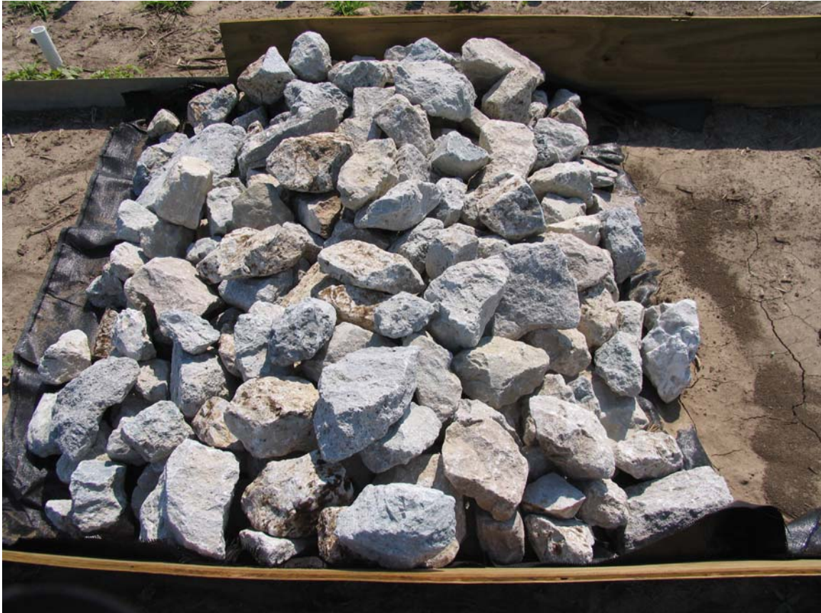
Figure 4.1. Riprap berm at field study site.
