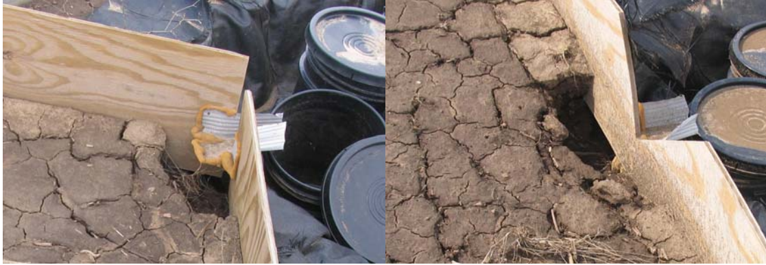
Figure 5.11. Washout and scour occurring around both end structures used on plots.
