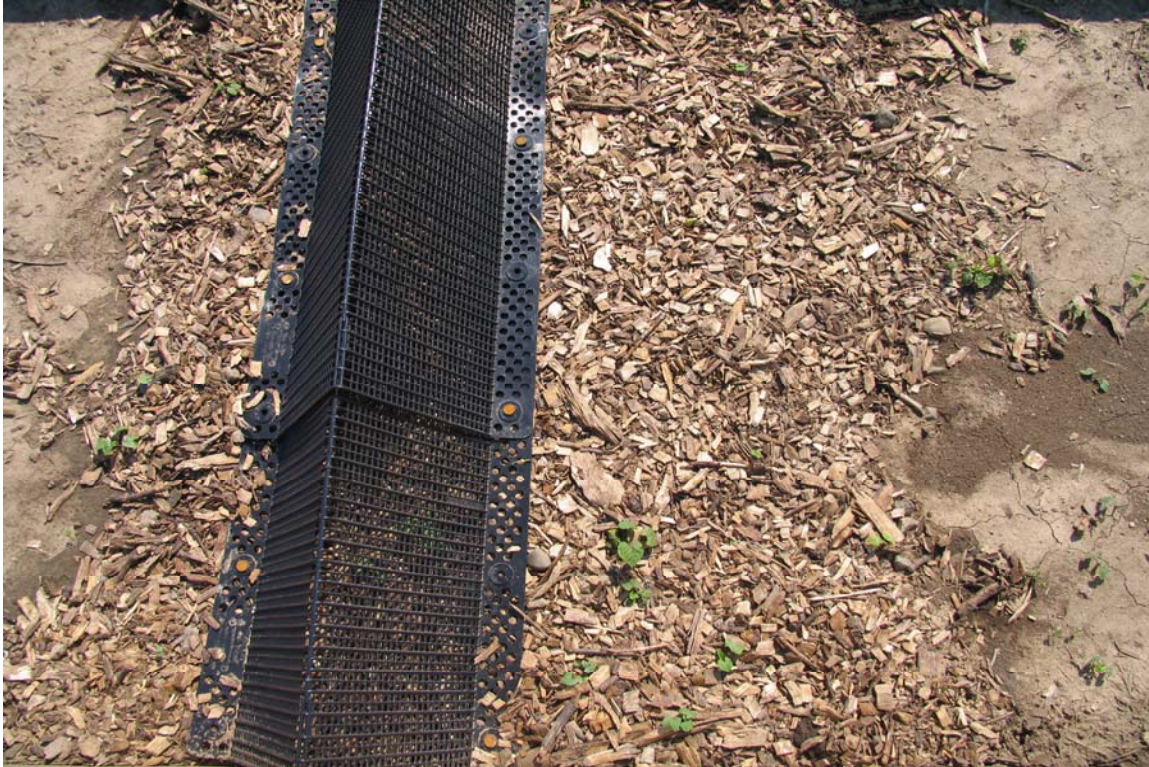
Figure 4.6. Plastic dam and compost blanket and field site.
