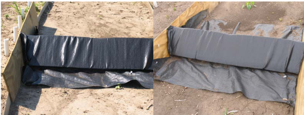
Figure 5.15. Undercutting of the geotextile common with the foam berm.
