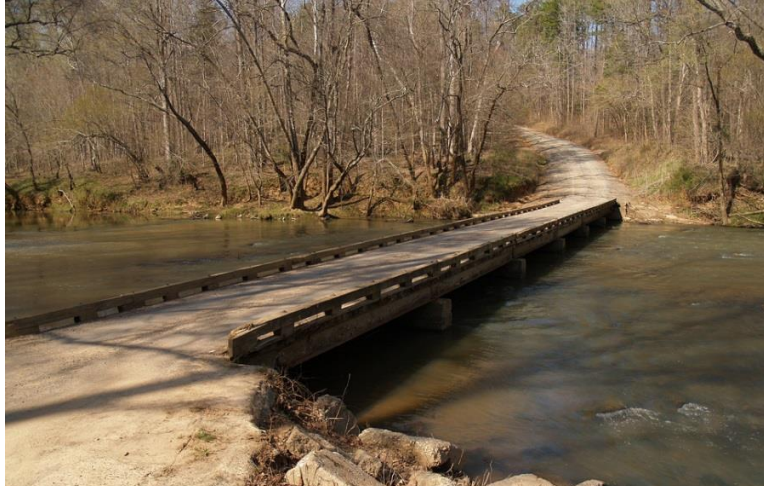
Figure 3.3: Low water bridge at Montgomery County, North Carolina (Filer, 2008).
