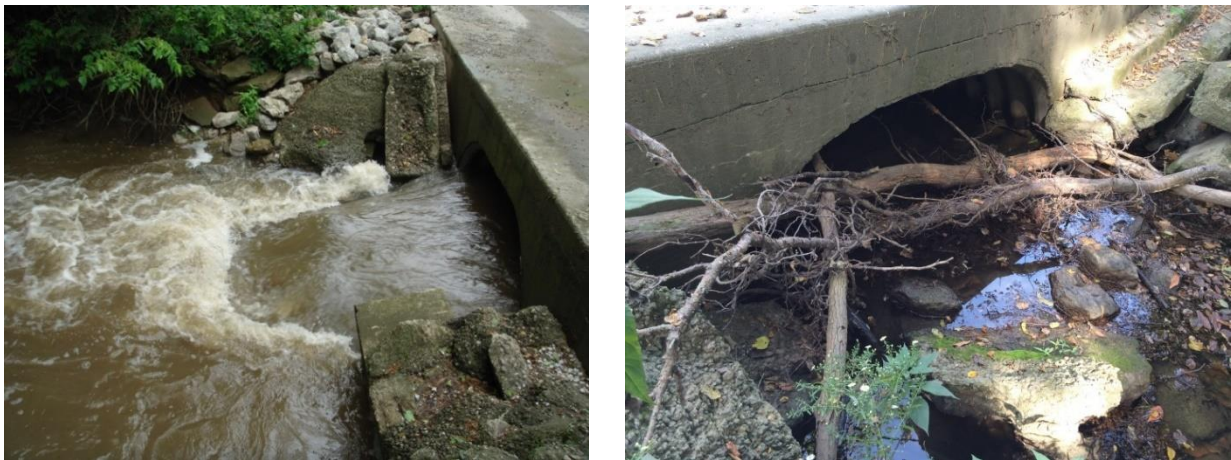
Figure 4.6: Edgar#1 LWC after a rainfall event (left), same LWC during dry months (right).
