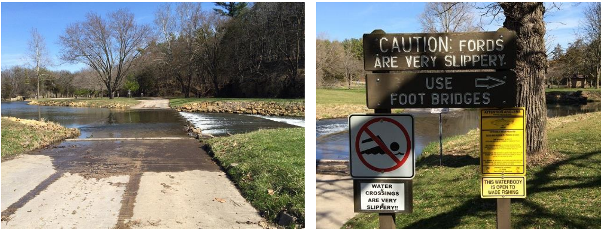
Figure 4.18: Low water crossing under study and warning sign.
