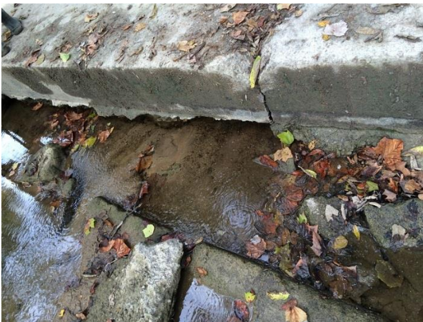
Figure 4.10: Low water crossing and the approach, Sediment deposition upstream, Undercutting on downstream end (clockwise direction from top).
